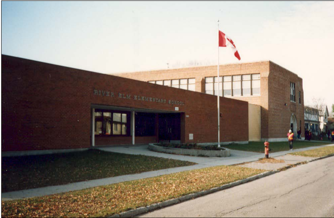
Front (north) and east façades, 1995
