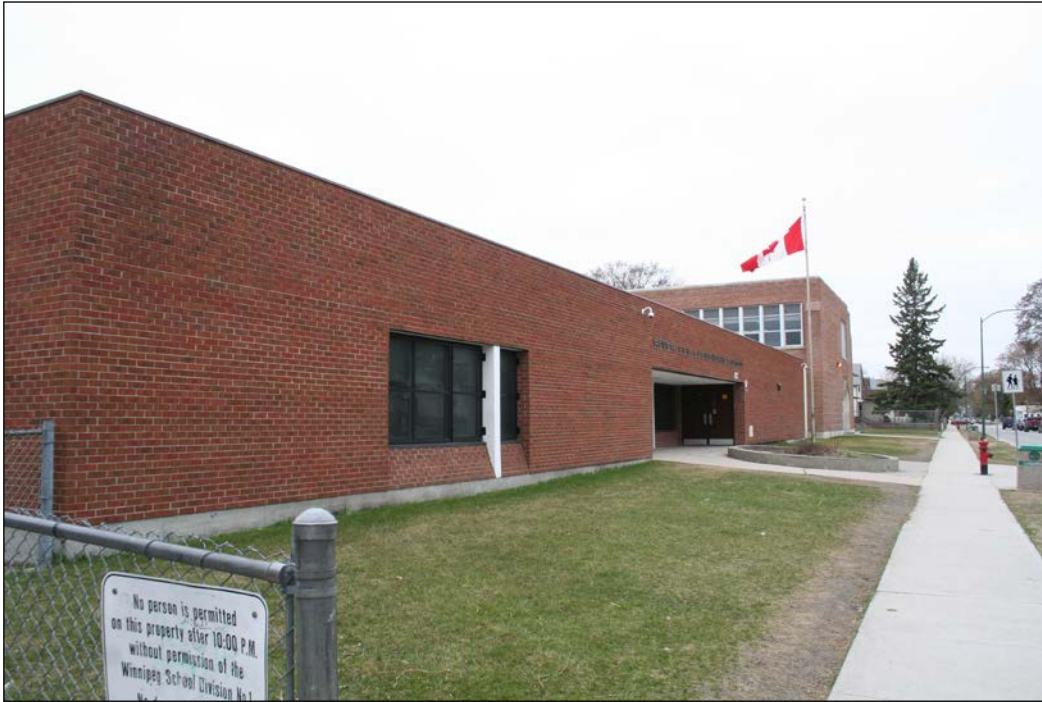
Front (north) and east façades, 2009
