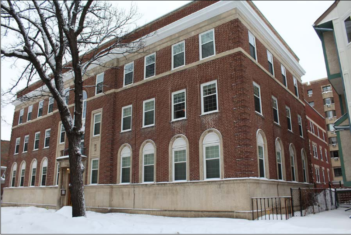
Plate 10 – Rossmore Apartments, 80 Roslyn Road, front (north) and west façades, 2106. ( M. Peterson, 2016. )
