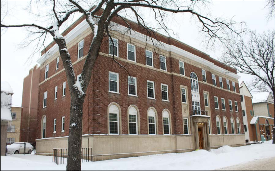
Plate 7 – Rossmore Apartments, 80 Roslyn Road, front (north) and east façades, 2106. ( M. Peterson, 2016. )
