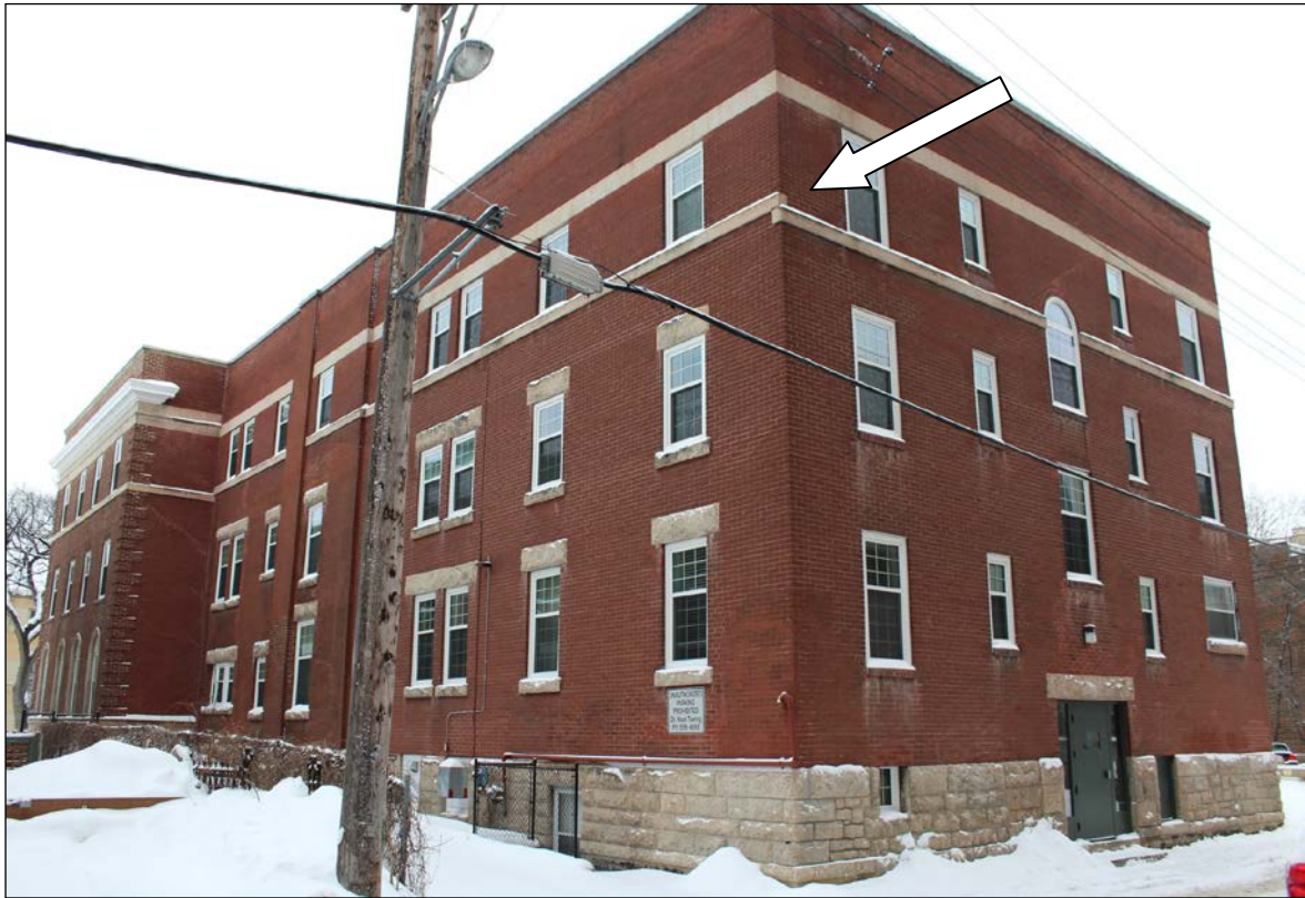
Plate 13 – Rossmore Apartments, 80 Roslyn Road, west and south façades of original and 1929 buildings, 2106. Note that the stone belt course does not meet perfectly at the southwest corner (arrow). (M. Peterson, 2016.)
