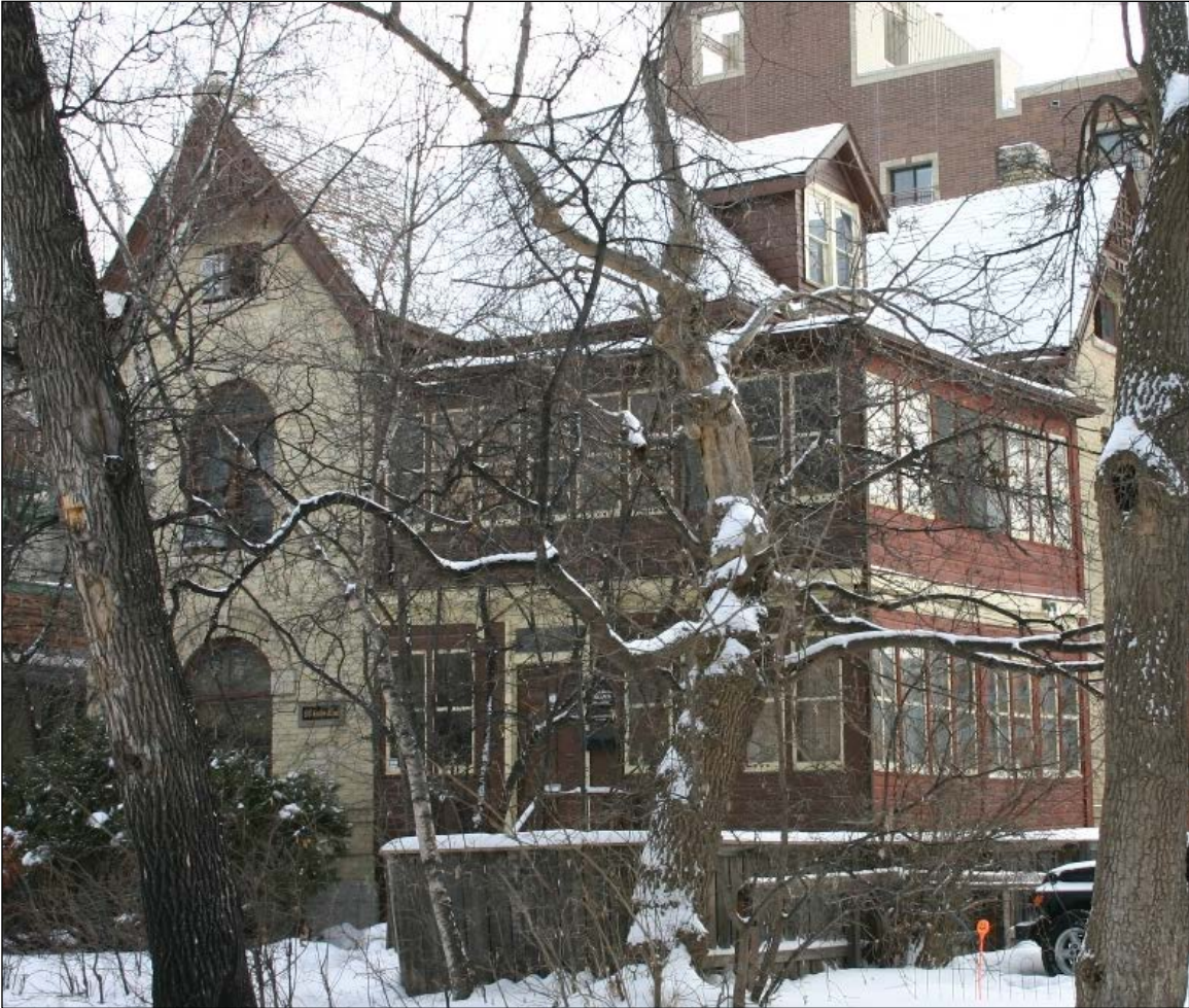
Plate 7 – Leslie Ironside House, 94 Roslyn Road, front (north) and west façades, 2010. ( M. Peterson, 2010. )
