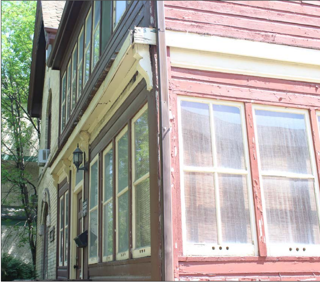
Plate 8 – Leslie Ironside House, 94 Roslyn Road, detail of front porch, 2018. ( M. Peterson, 2018. )
