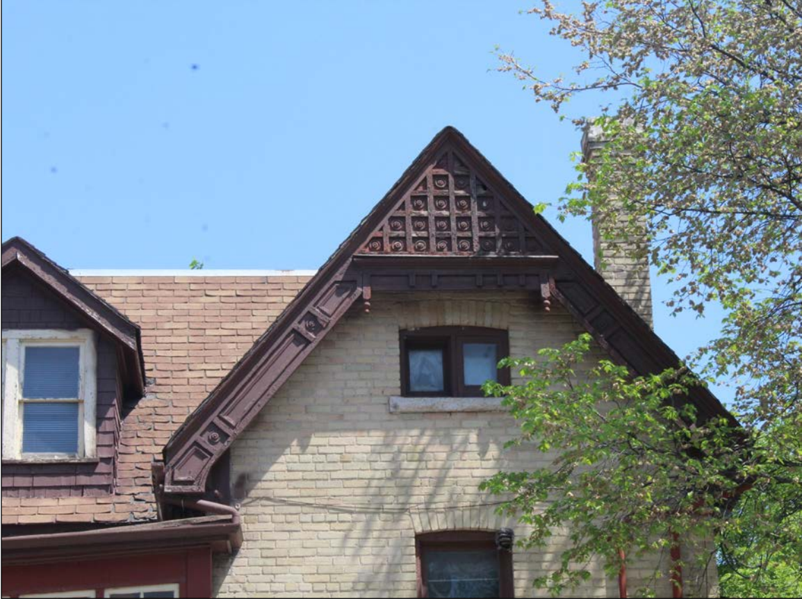
Plate 10 – Leslie Ironside House, 94 Roslyn Road, bargeboard on the west façade, 2018. ( M. Peterson, 2018. )
