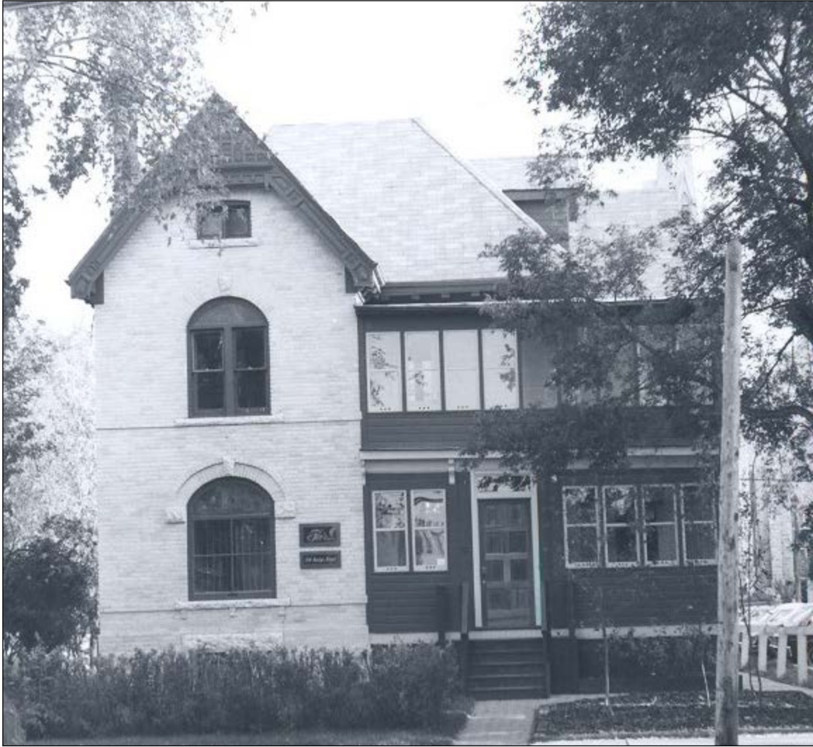
Plate 13 – Leslie Ironside House, 94 Roslyn Road, front (north) façade, 1978. ( City of Winnipeg. )
