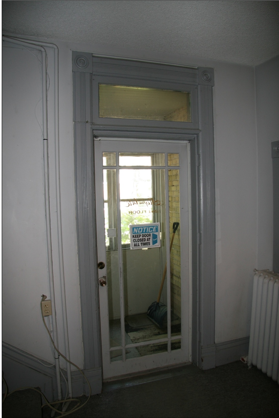
Plate 15 – Leslie Ironside House, 94 Roslyn Road, front entrance with transom and wood trim, 2018. (M. Peterson, 2018.)
