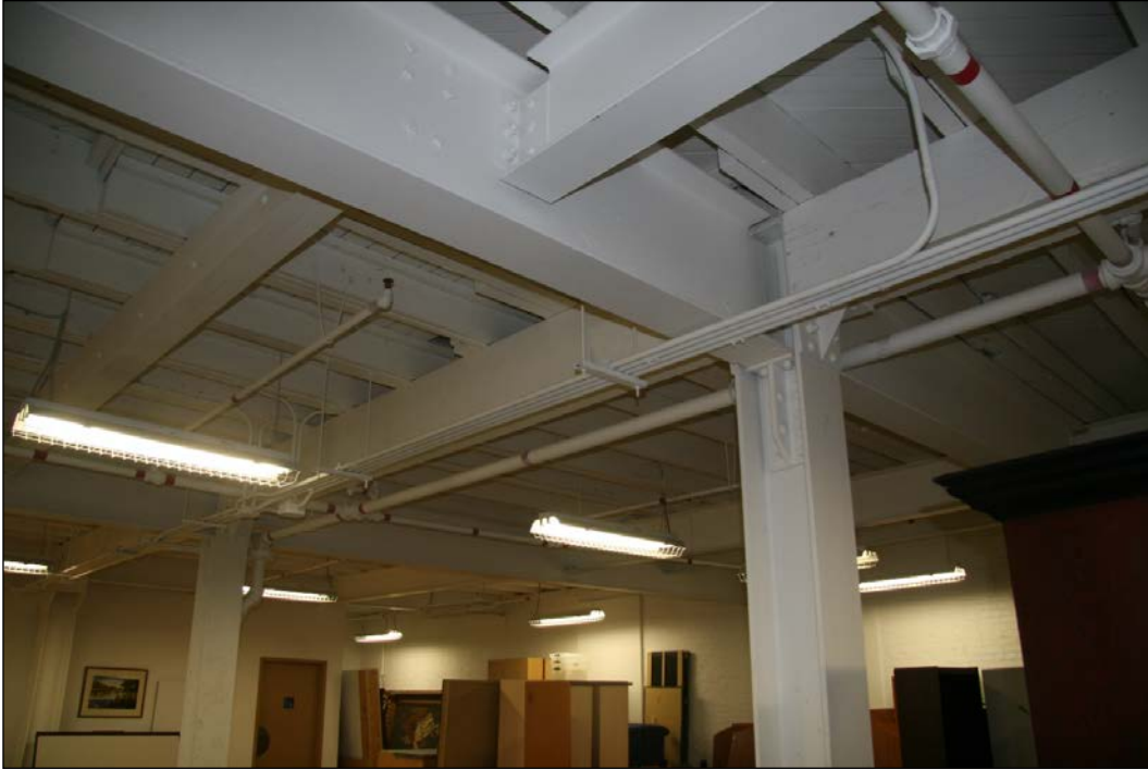
Plate 17 – Paulin-Chambers Building, 311 Ross Avenue, first floor, steel support system, 2018. (M. Peterson, 2018.)
