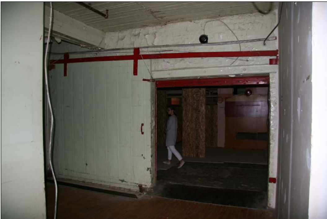
Plate 20 – Paulin-Chambers Building, 311 Ross Avenue, metal-clad fire door, 4 th floor, 2018. (M. Peterson, 2018.)
