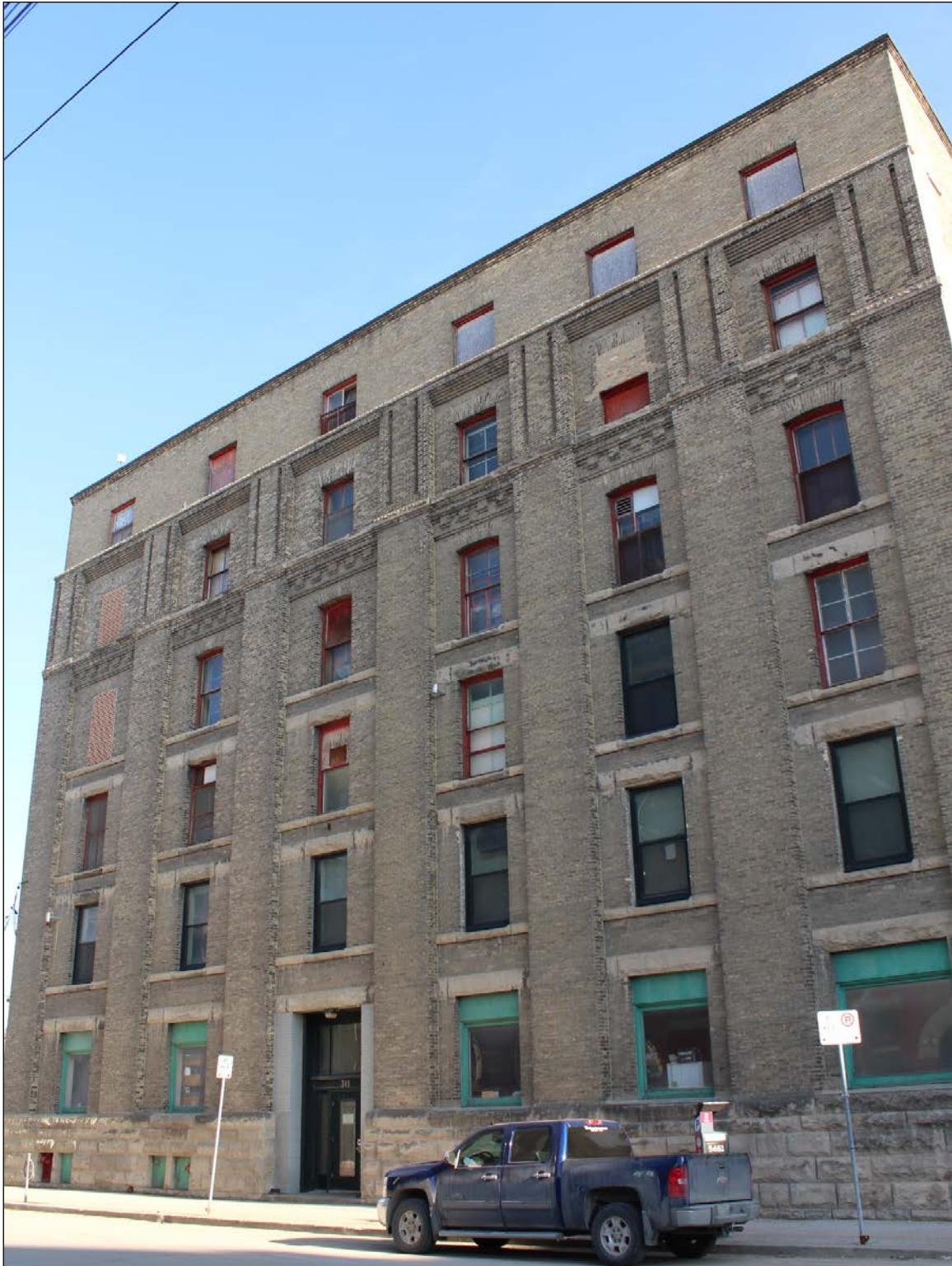
Plate 9 – Paulin-Chambers Building, 311 Ross Avenue, front (south) façade, 2016. (M. Peterson, 2016.)
