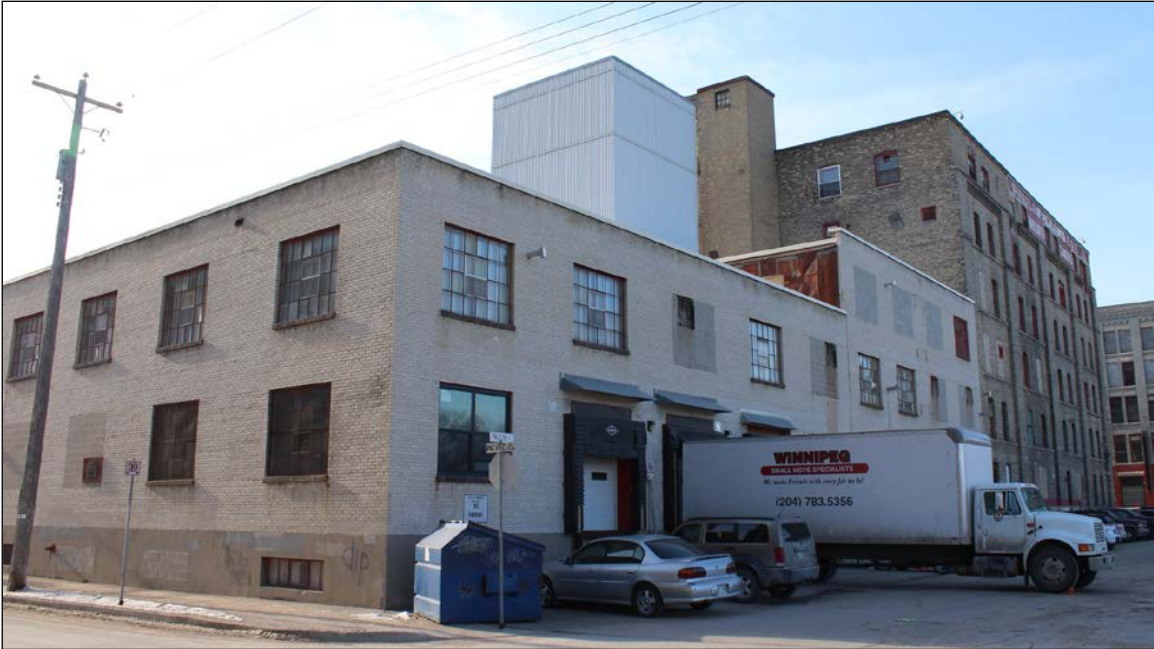
Plate 14 – Paulin-Chambers Building, 311 Ross Avenue, rear addition, north and west façades, 2016. (M. Peterson, 2016.)
