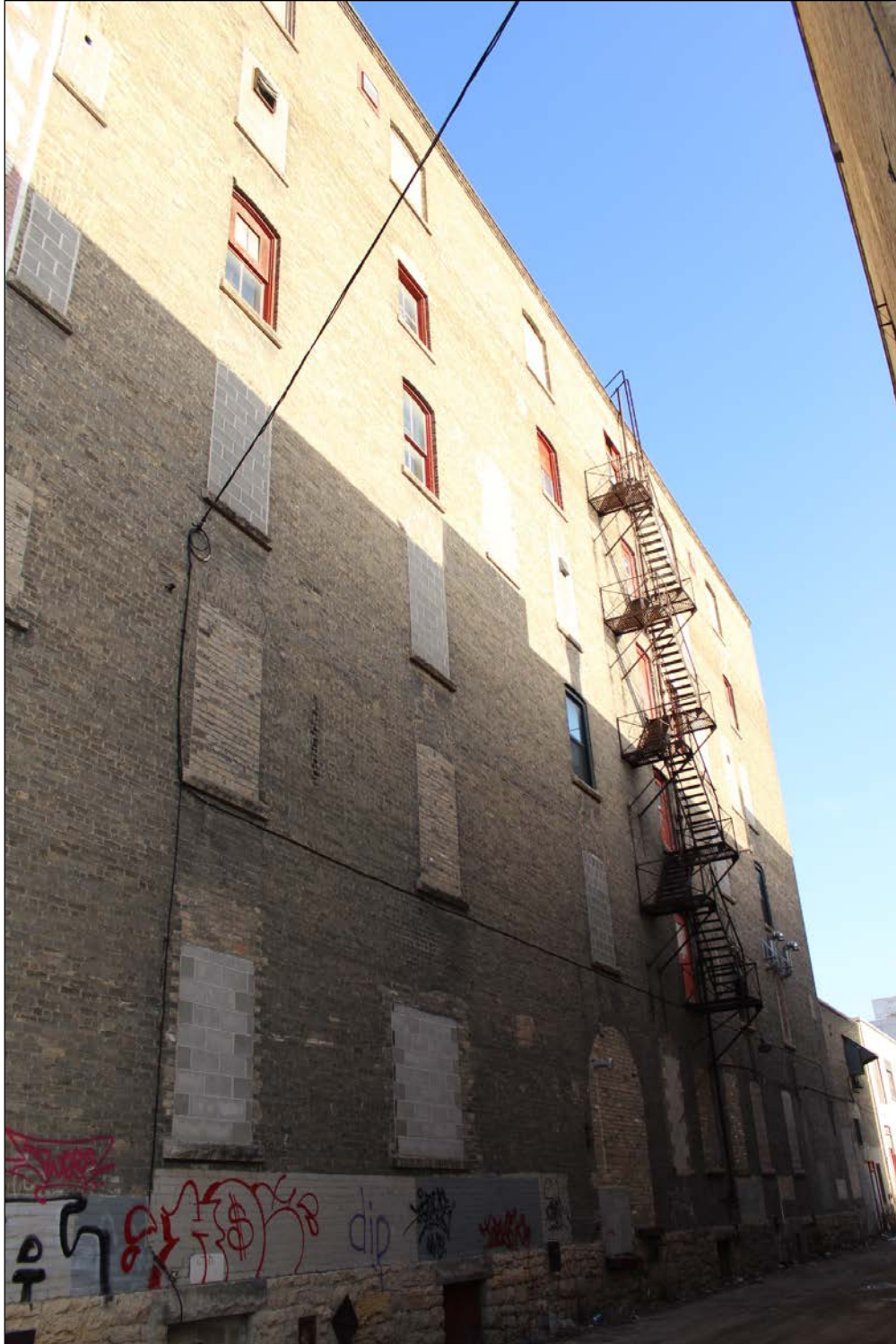
Plate 12 – Paulin-Chambers Building, 311 Ross Avenue, east façade, 2016. (M. Peterson, 2016.)
