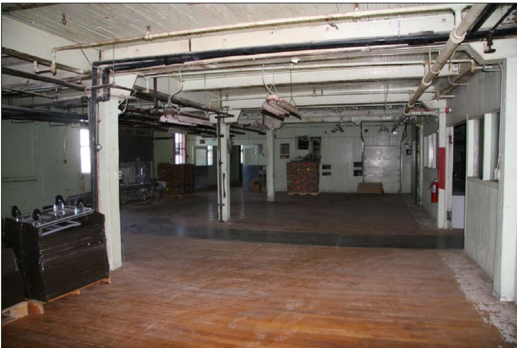
Plate 18 – Paulin-Chambers Building, 311 Ross Avenue, mill construction, 5 th floor, 2018. (M. Peterson, 2018.)
