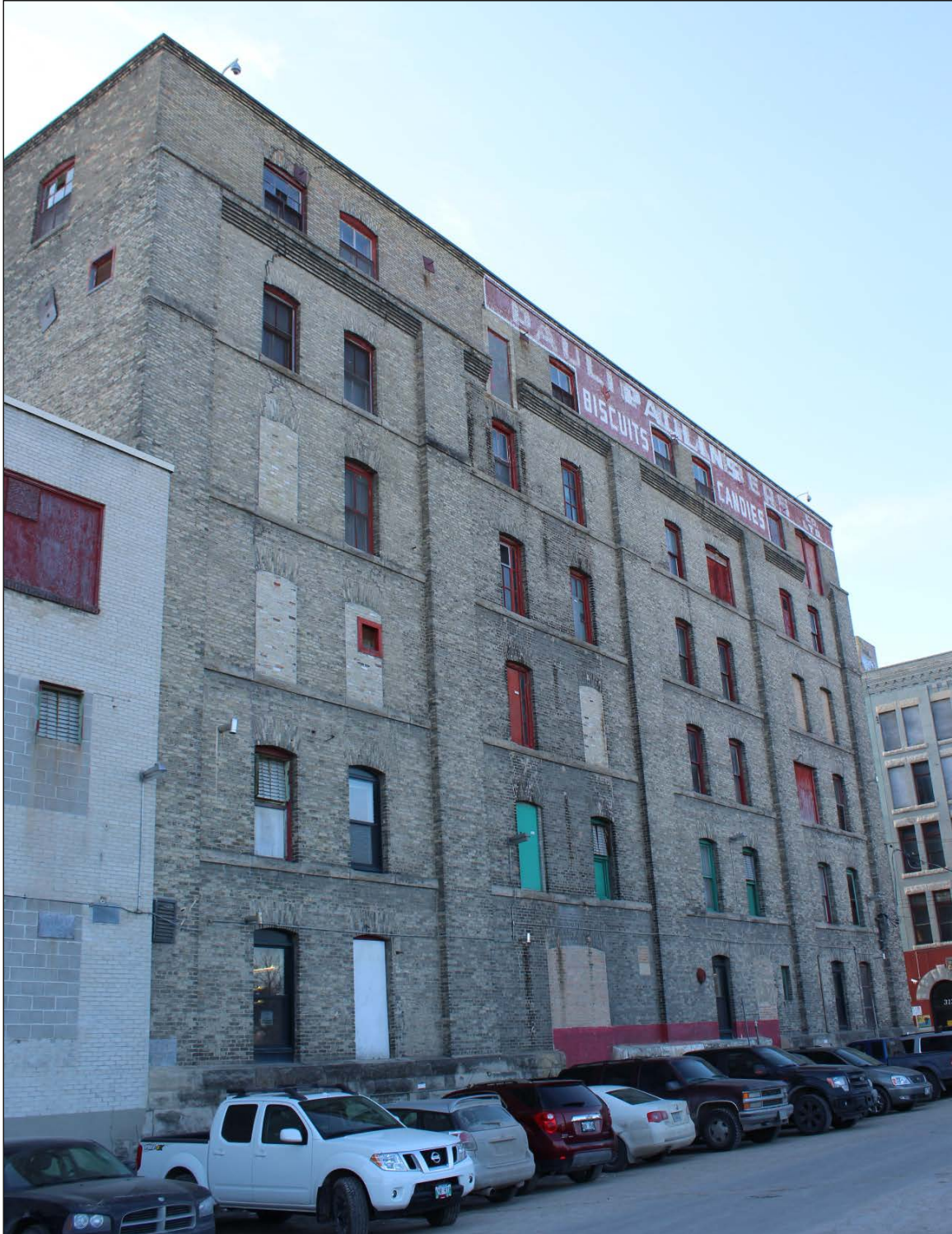
Plate 11 – Paulin-Chambers Building, 311 Ross Avenue, west façade, 2016. (M. Peterson, 2016.)
