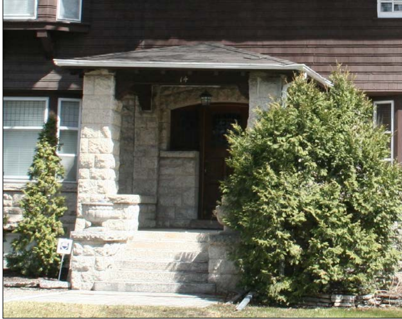
Front (west) façade detail, 2009
