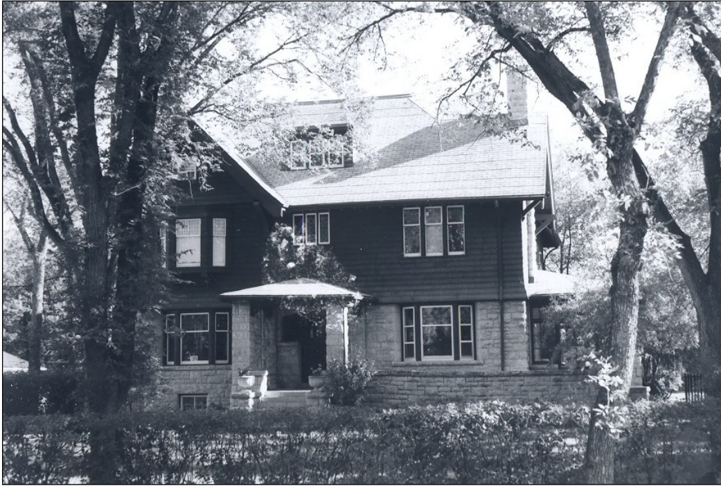
Front (west) façade, 1978
