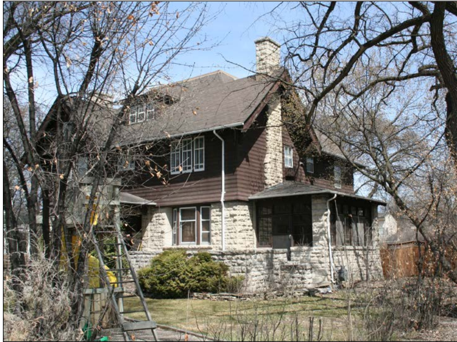
Front (west) and south façades, 2009
