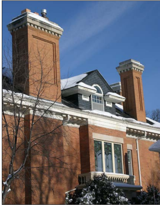
South façade detail, 2009
