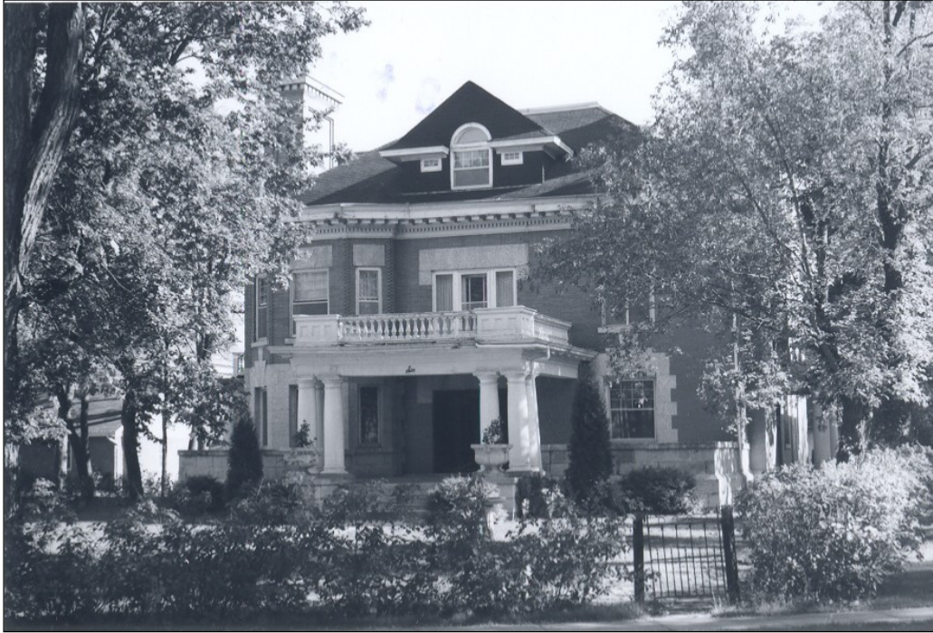
Front (west) façade, 1978
