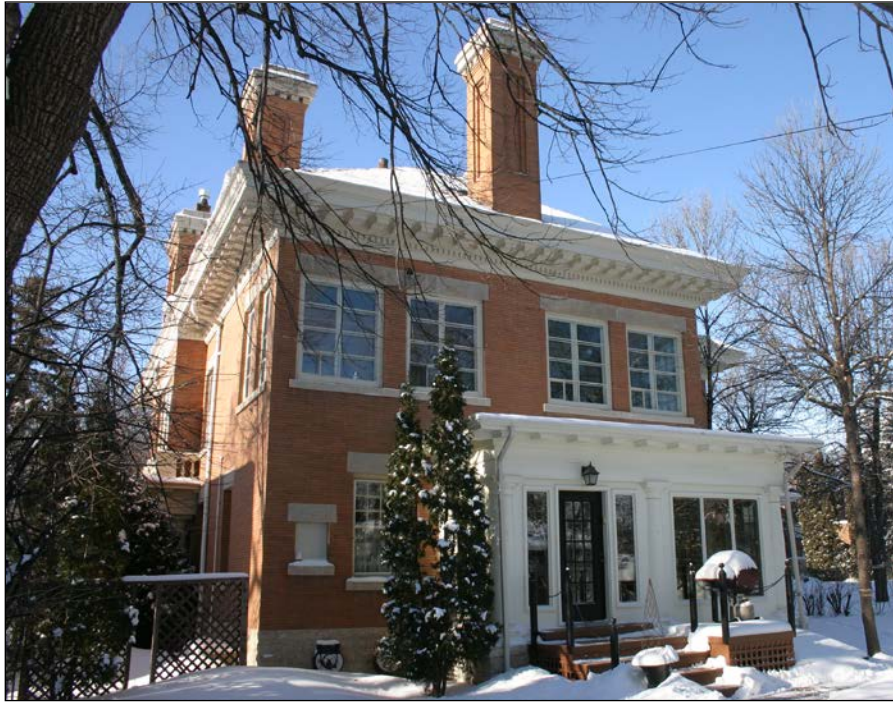
Rear (east) and south façades, 2009
