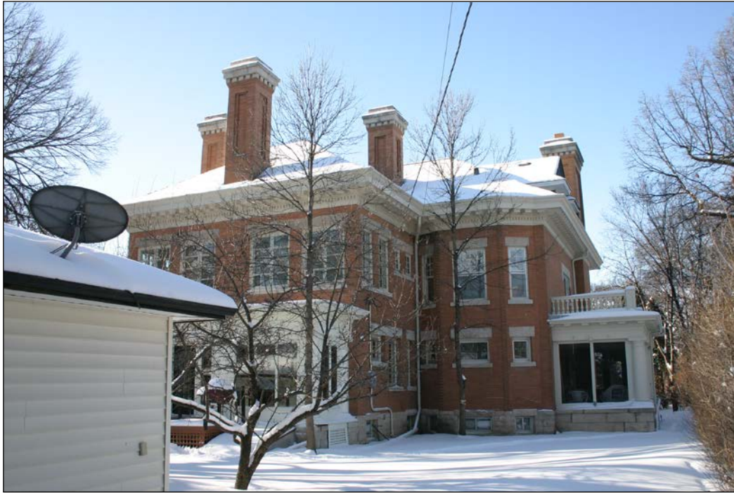
Rear (east) and north façades, 2009
