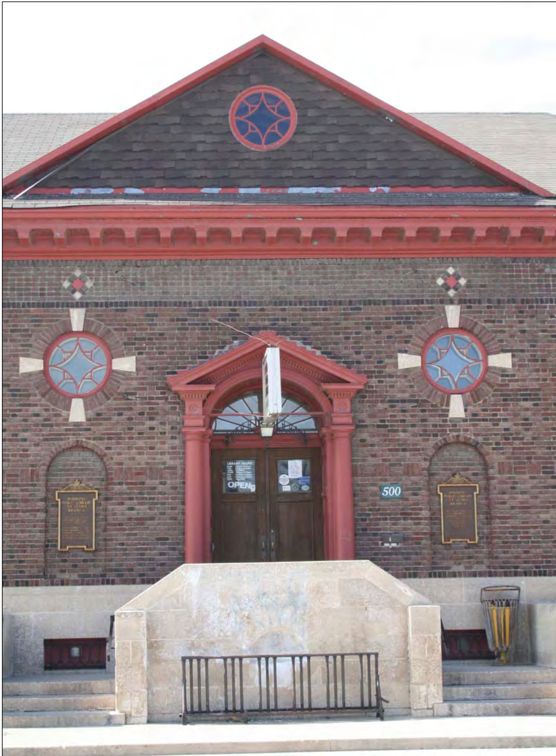
Plate 4 – St. John’s Library, 500 Salter Street, front (east) façade detail, 2010. (M. Peterson, 2010. )
