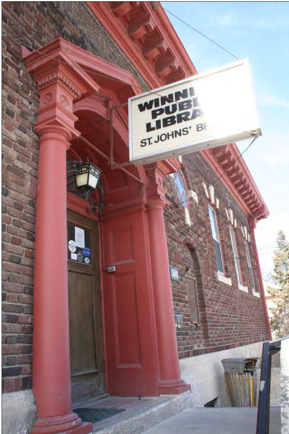
Plate 5 – St. John’s Library, 500 Salter Street, front (east) façade entrance, 2010. ( M. Peterson, 2010. )
