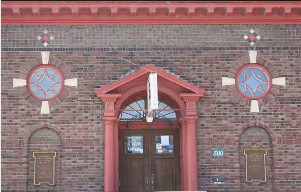
Plate 7 – St. John’s Library, 500 Salter Street, front (east) façade detail, 2010. ( M. Peterson, 2010. )
