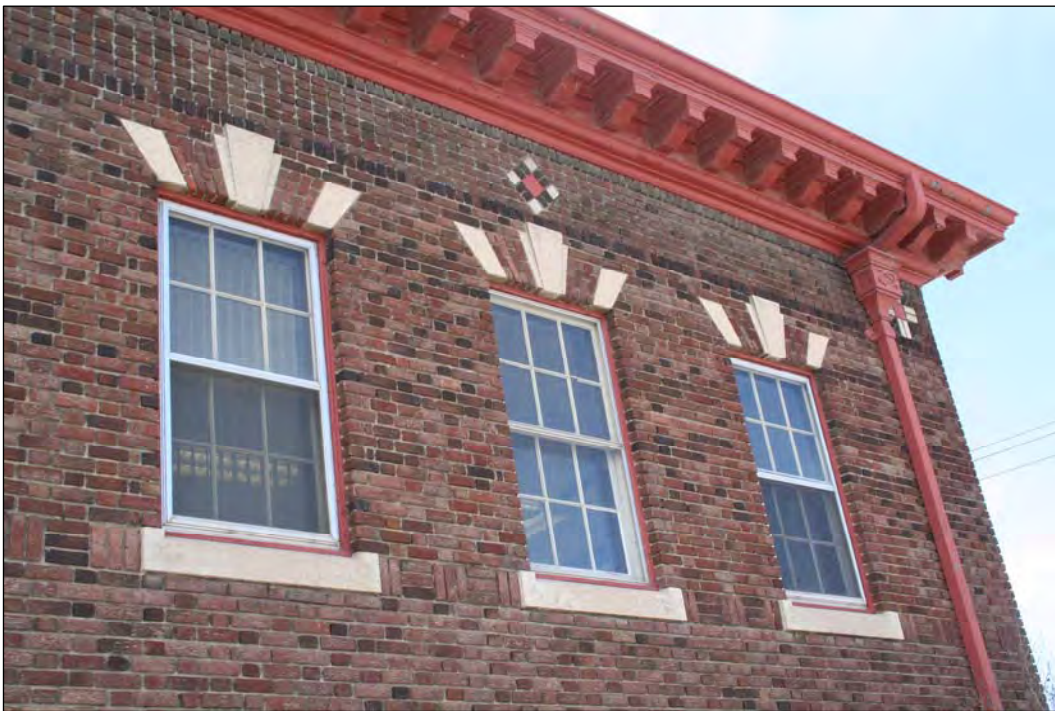
Plate 8 – St. John’s Library, 500 Salter Street, front (east) façade detail, 2010. ( M. Peterson, 2010. )
