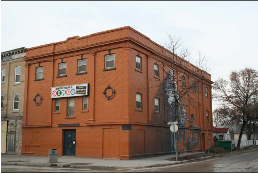
Front (south) and east façades, 2008
