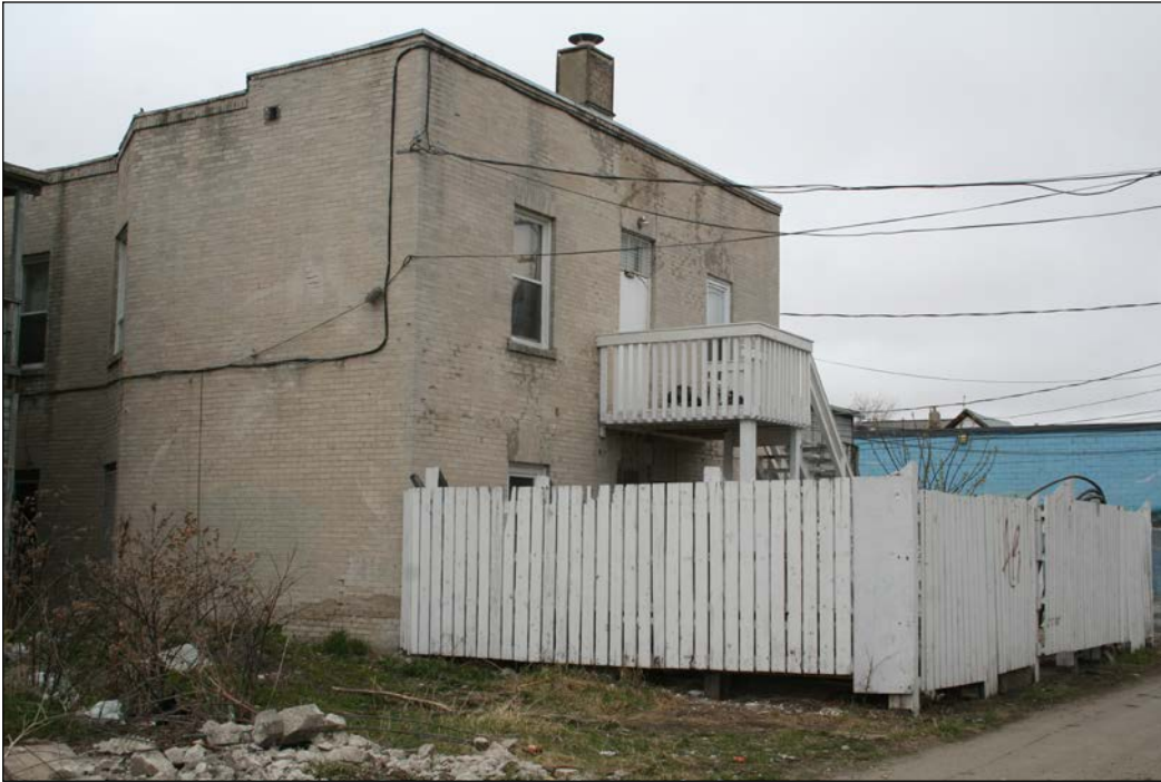
Rear (north) and east façades, 2009
