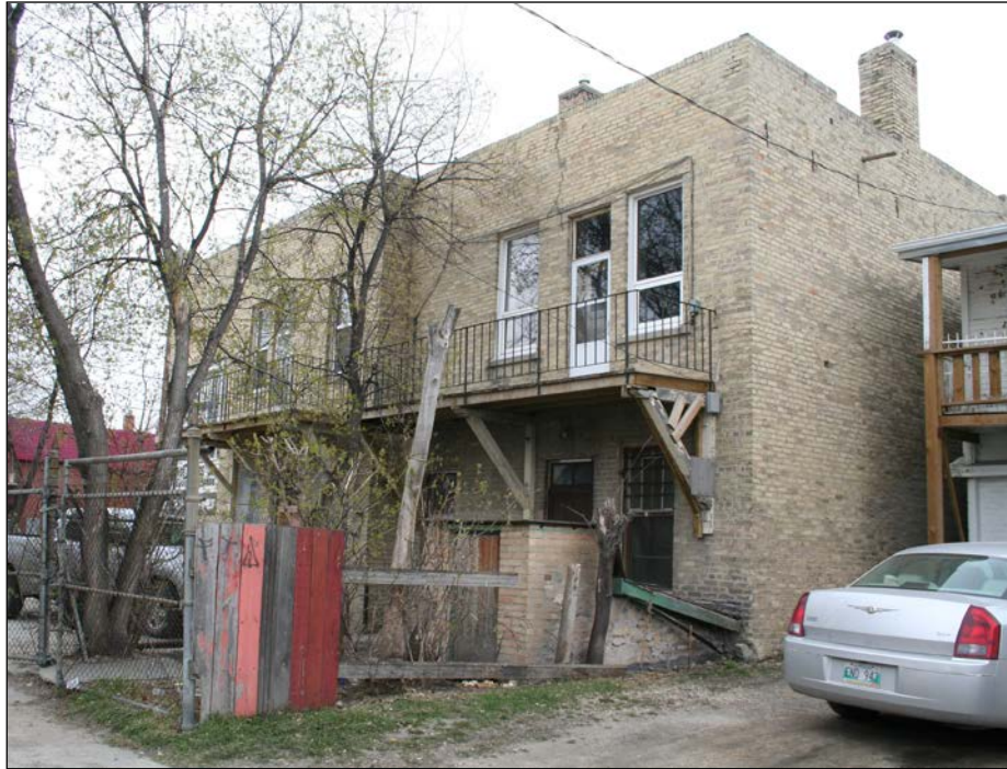
Rear (south) and east façades, 2009
