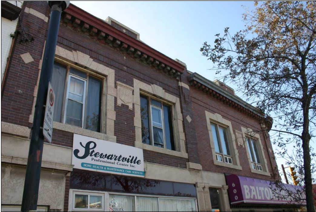
North façade detail, 2009
