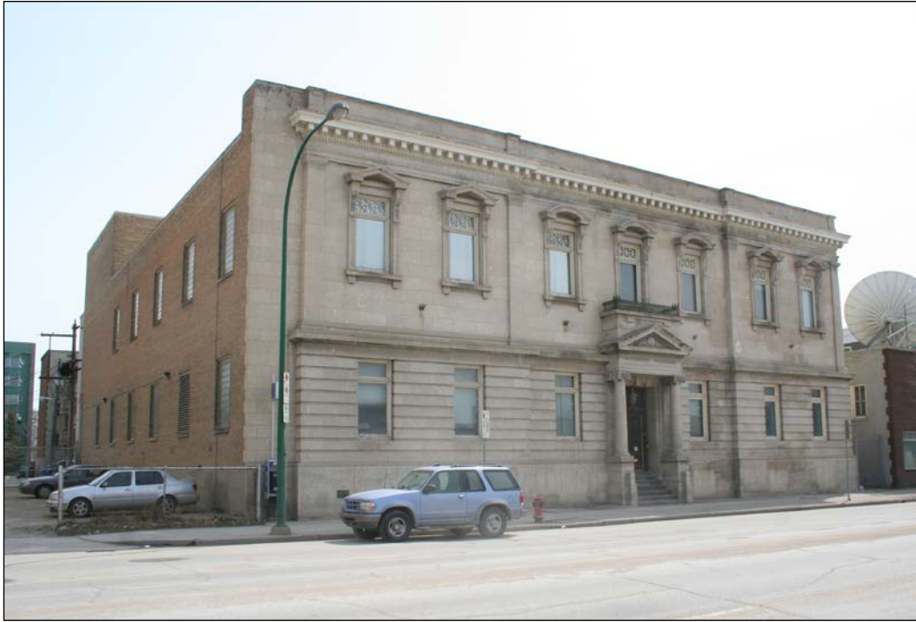
Front (west) and north façades, 2009
