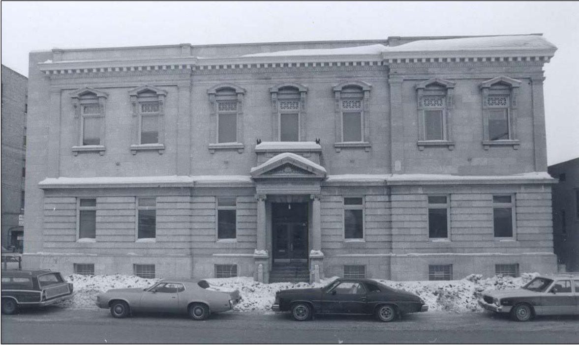
Front (west) façade, 1978
