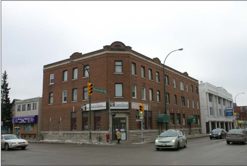
Front (west) and north façades, 2009
