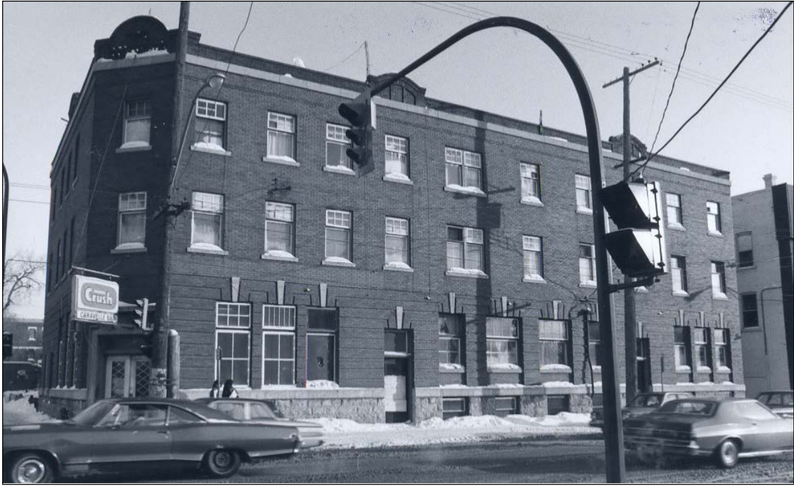
Front (west) and north façades, 1978
