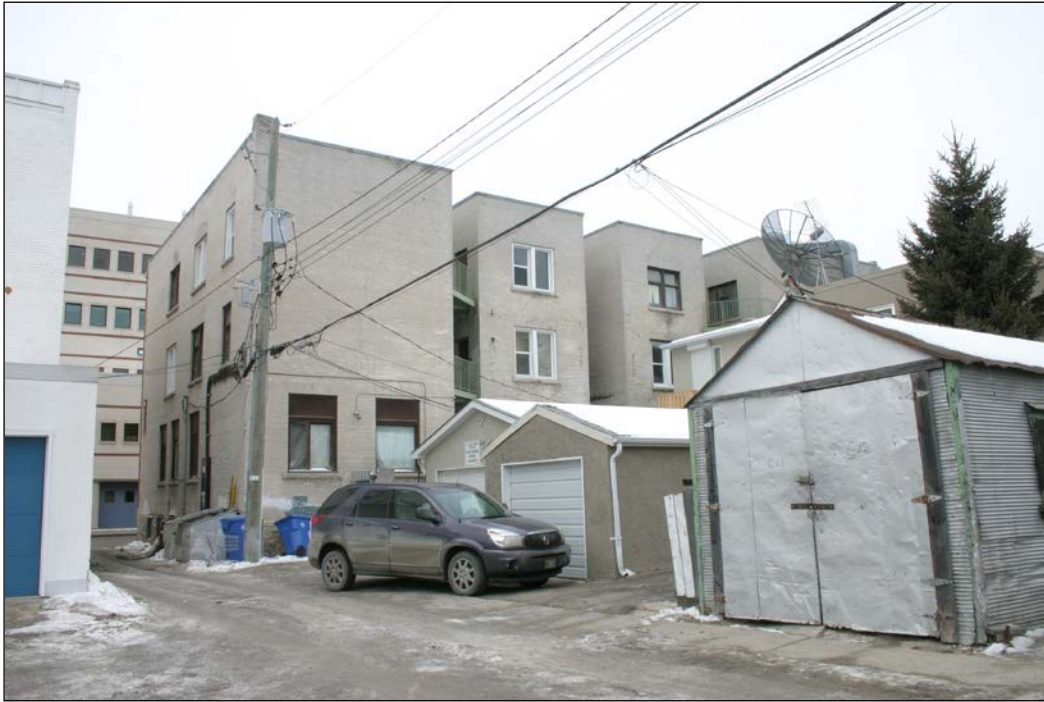
Rear (east) and south façades, 2009
