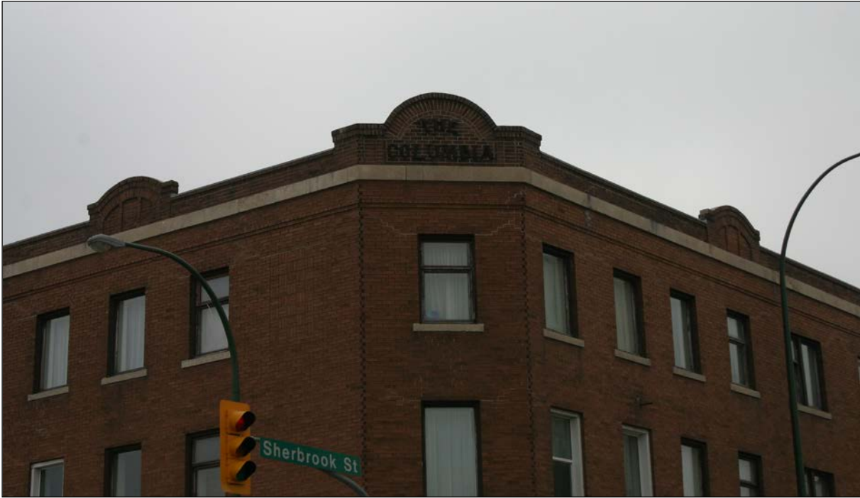
Northwest corner detail, 2009
