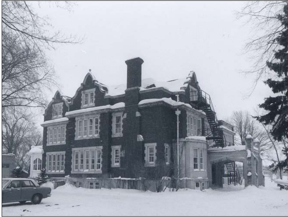
Front (west) and north façades, 1978
