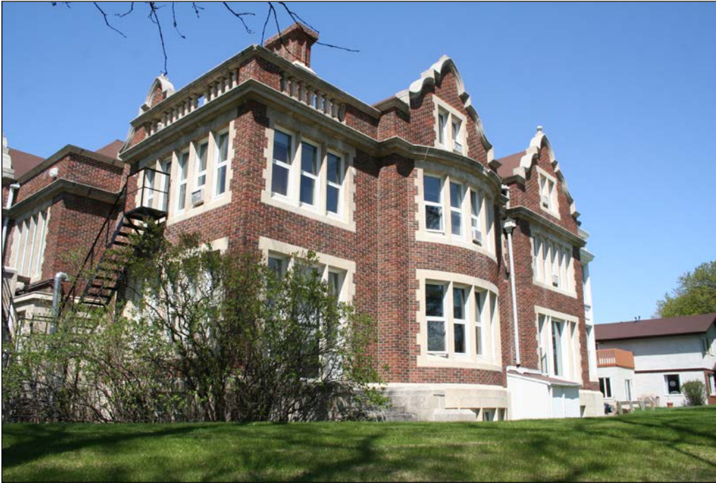
Rear (east) and south façades, 2009
