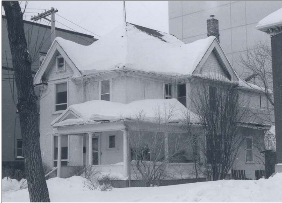
Front (east) and north façades, 1978
