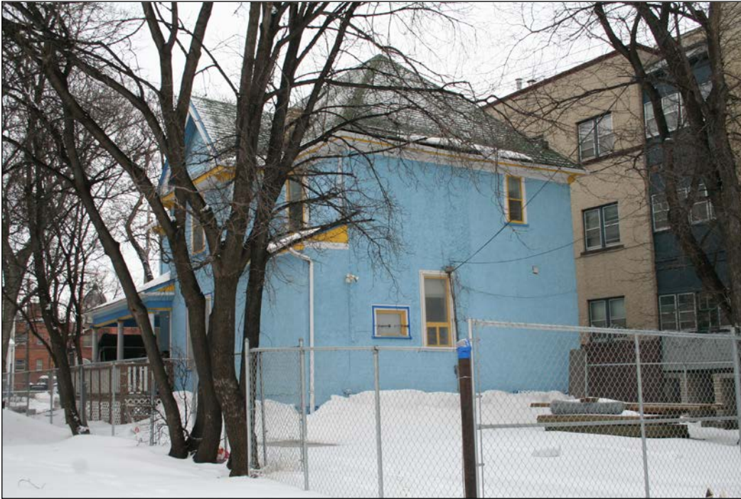
Rear (west) and north façades, 2009
