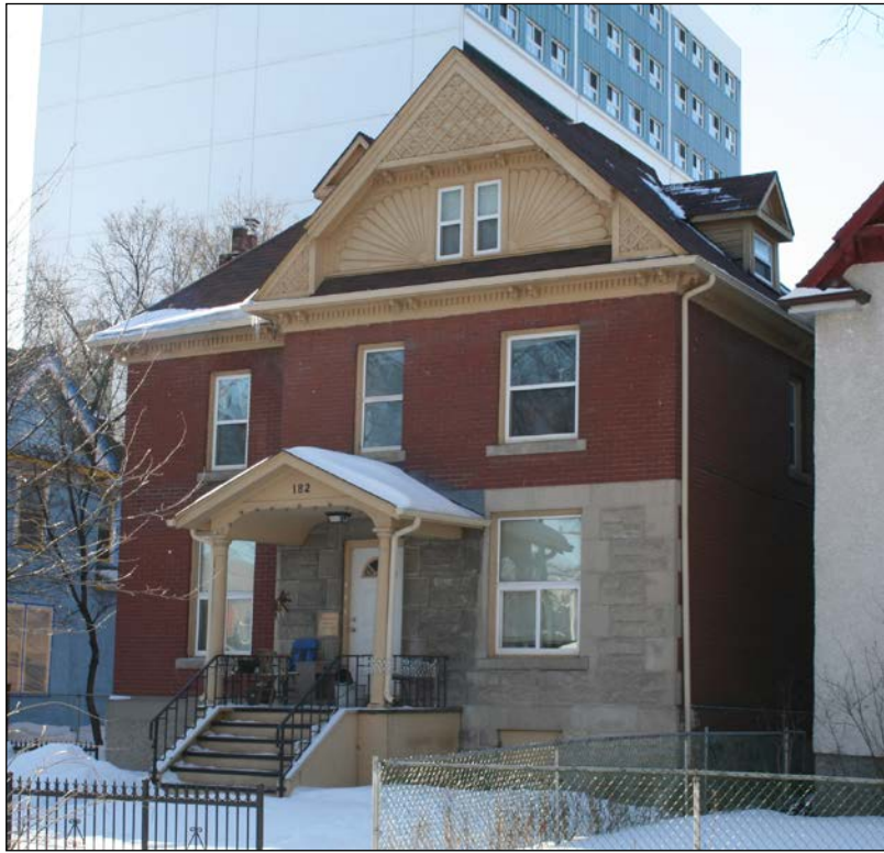
182 SPENCE STREET JOHN HAMILTON PARKHILL HOUSE
