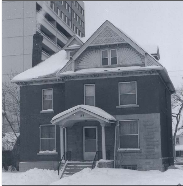
Front (east) façade, 1978
