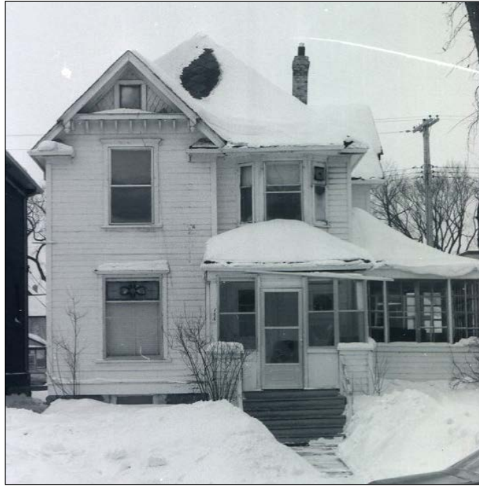
Front (east) façade, 1978
