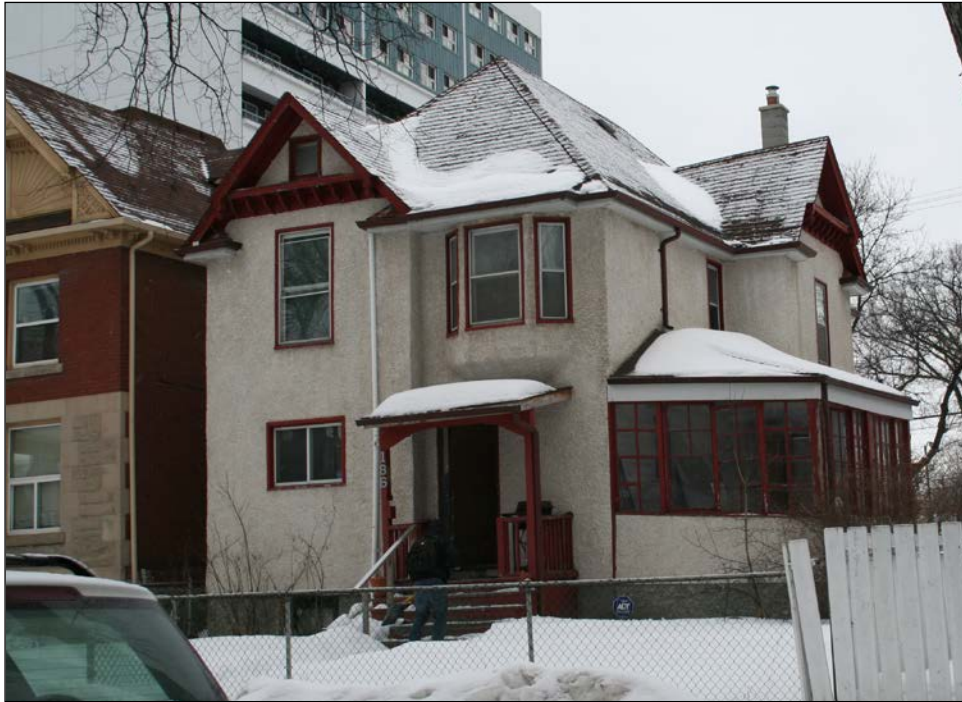
Front (east) and north façades, 2009
