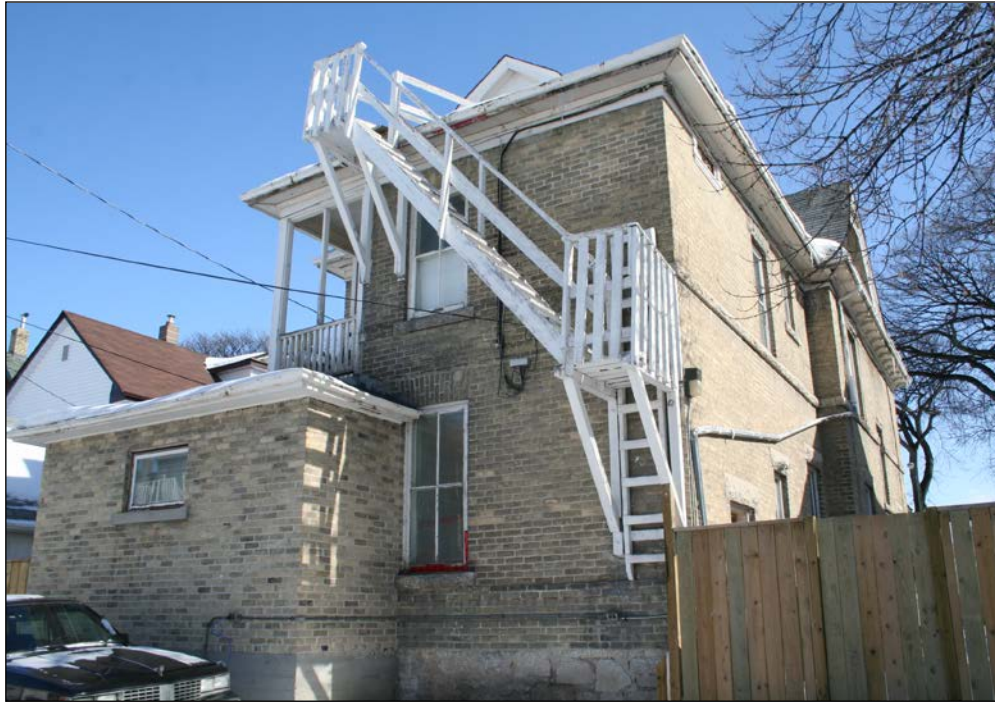
Rear (west) and south façades, 2009
