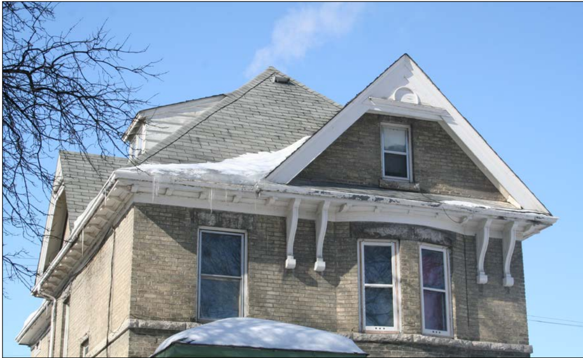
Front (east) façade detail, 2009
