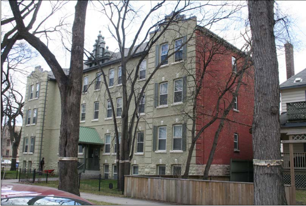
East and north façades, 2009
