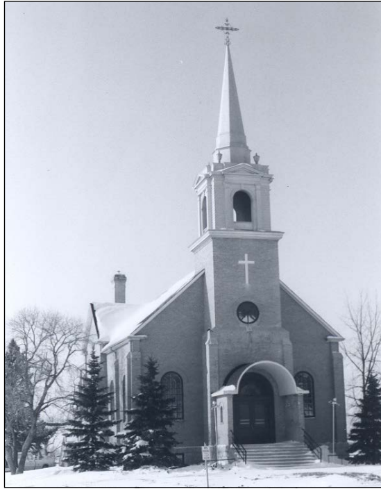
Front (east) façade, 1978
