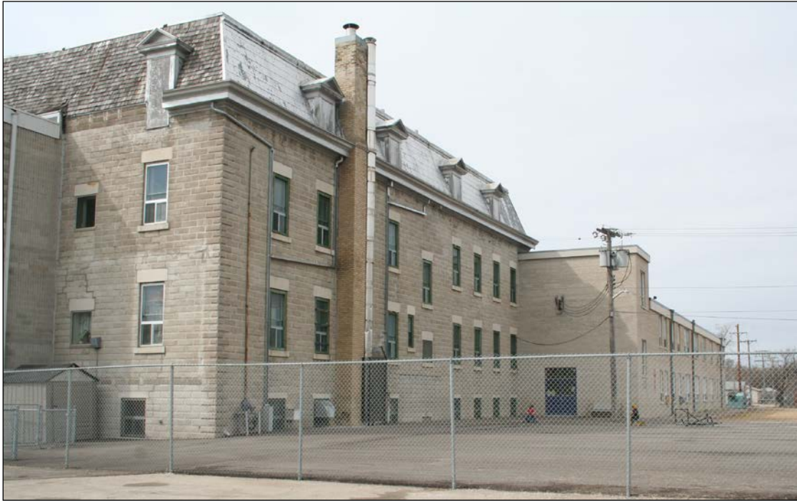
Rear (east) and south façades, 2009
