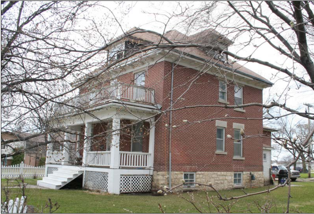
Front (east) and north façades, 2009
