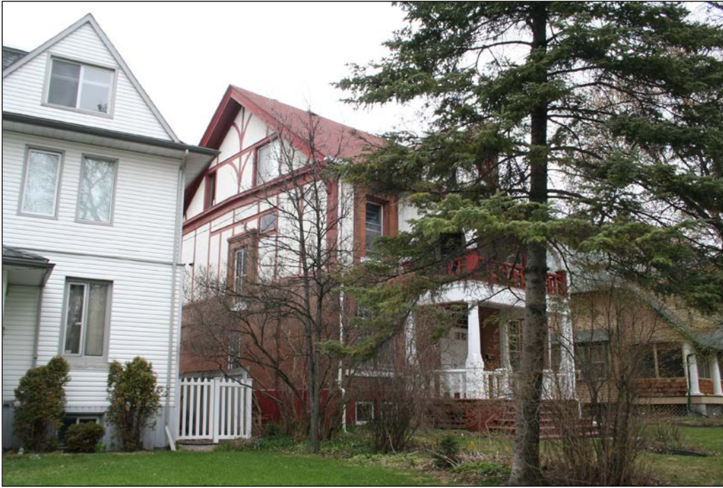
Front (east) and south façades, 2009
