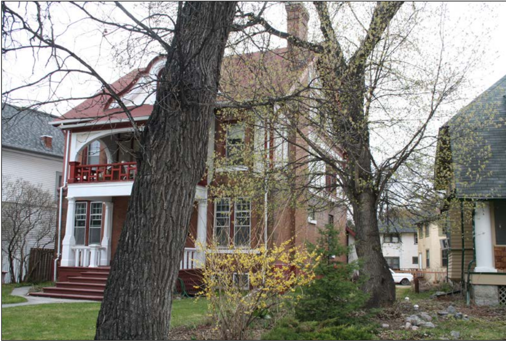
Front (east) and north façades, 2009
