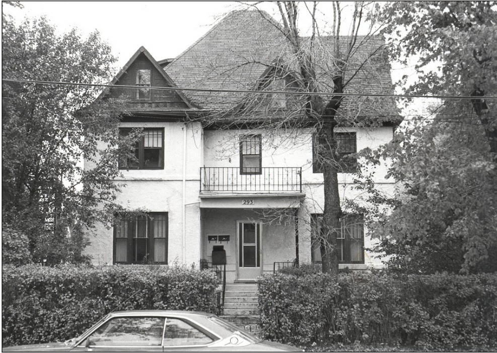
Front (south) façade, 1978
