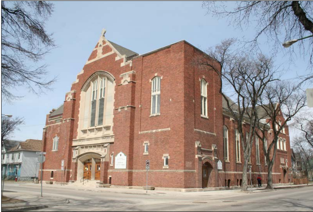
Front (south) and east façades, 2009
