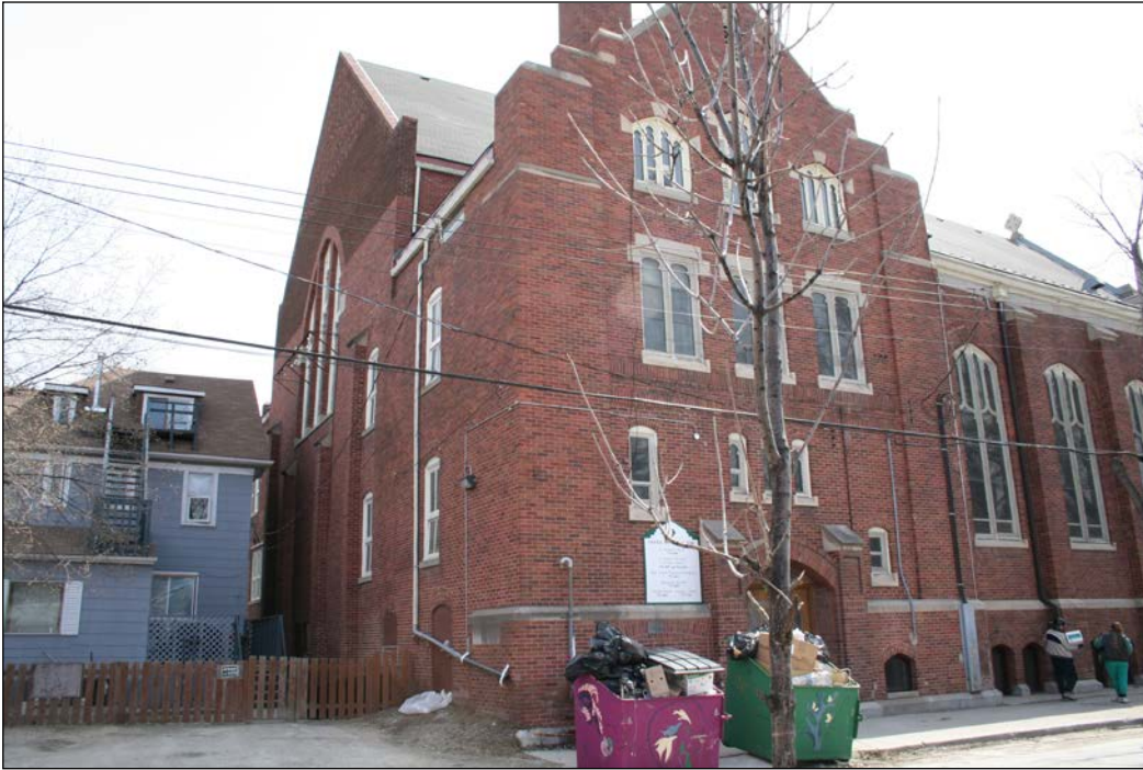
Rear (north) and west façades, 2009
