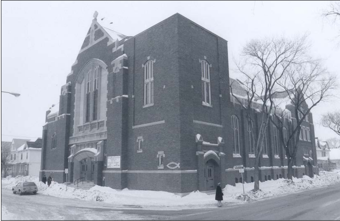
Front (south) and east façades, 1978
