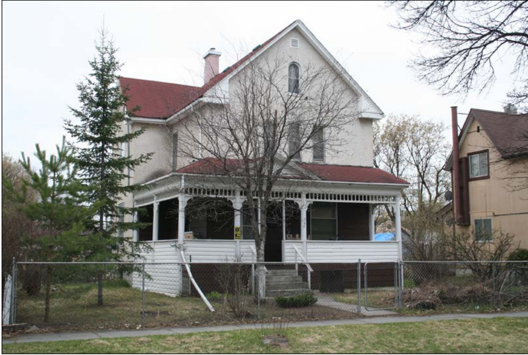
Front (north) and east façades, 2009
