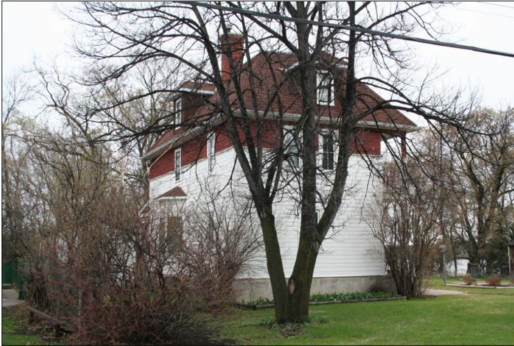
South and west façades, 2009
