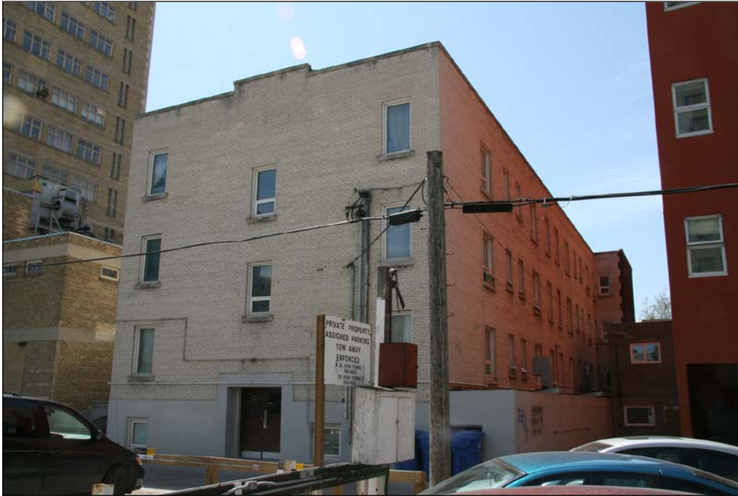
Rear (east) and north façades, 2007
