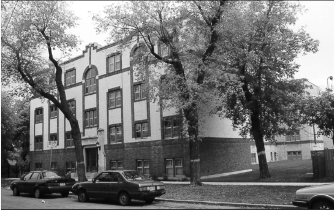
Plate 8 – Wiltshire Apartments, 30 Spence Street, front (east) façade. ( Murray Peterson, 1996. )
