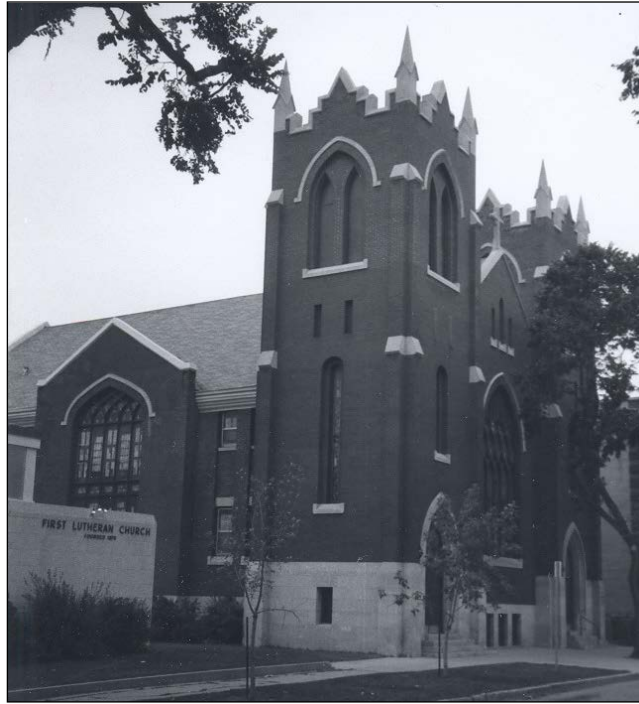
Front (east) and south façades, 1978
