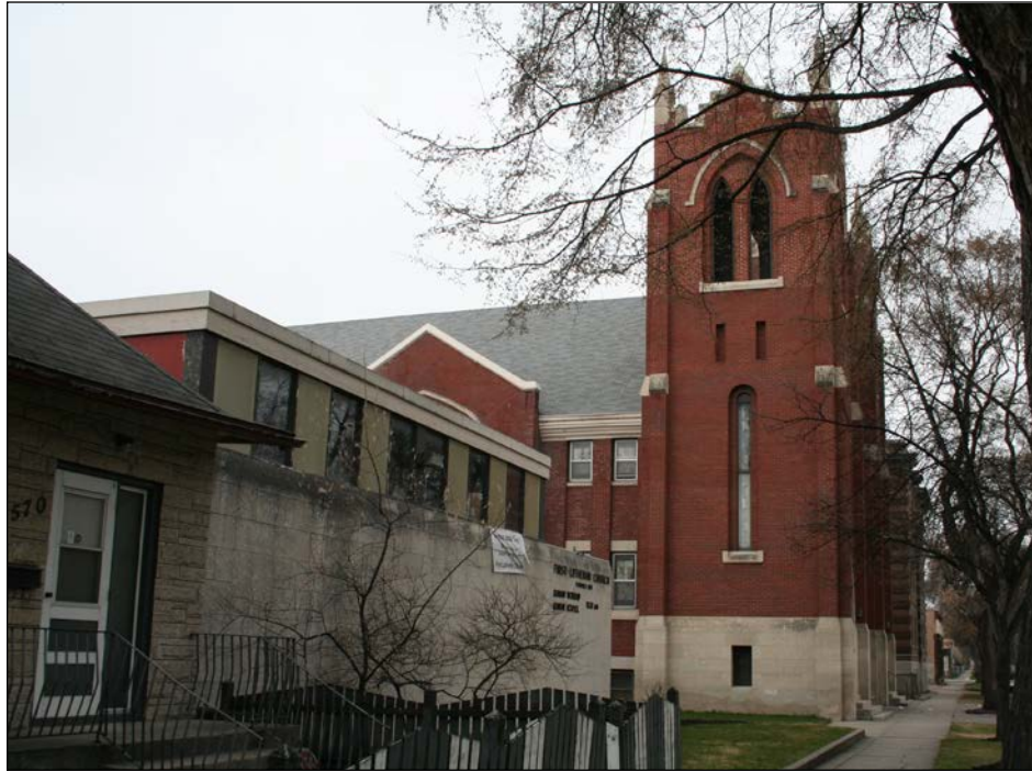
Front (east) and south façades, 2009
