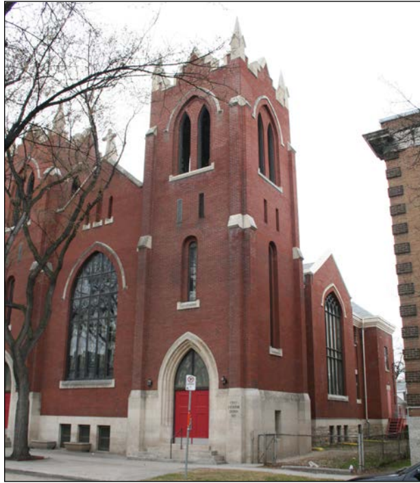
Front (east) and north façades, 2009
