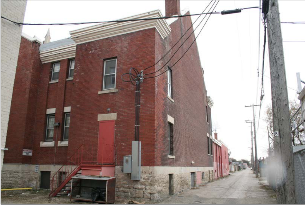
Rear (west) and north façades, 2009
