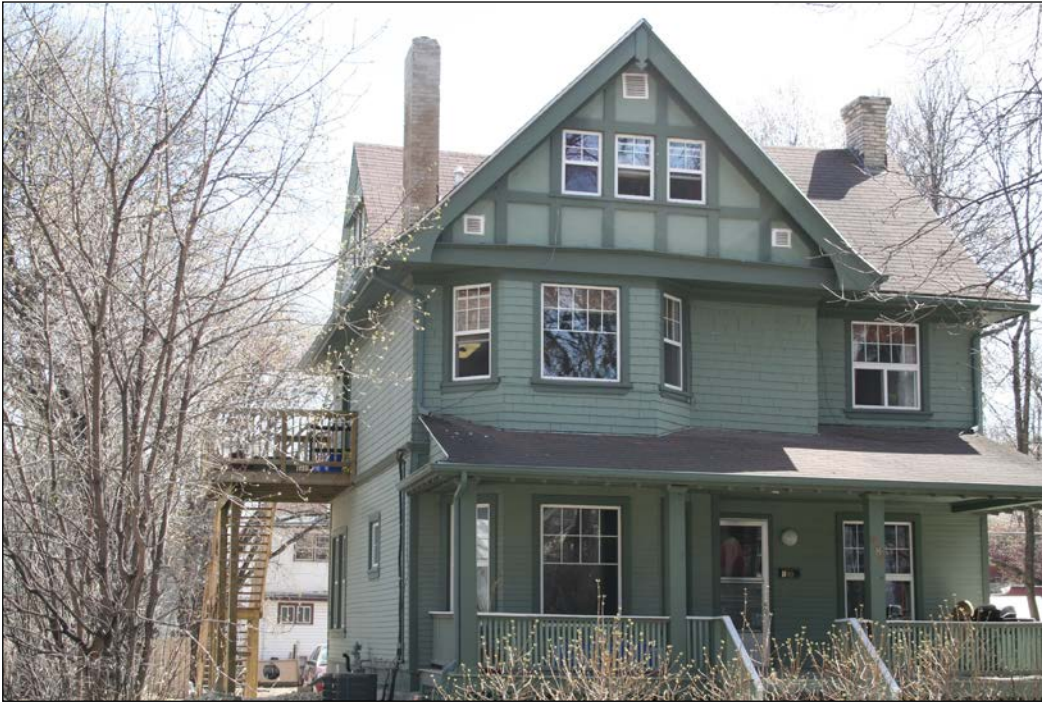
Front (north) and east façades, 2009
