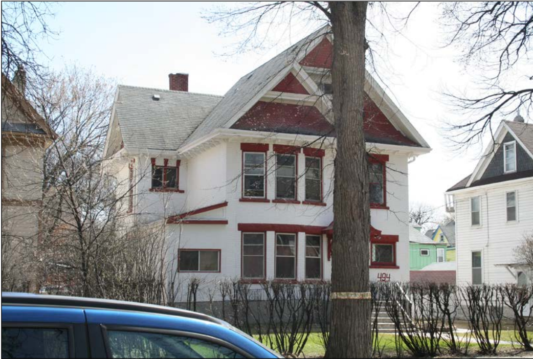
Front (north) and east façades, 2009
