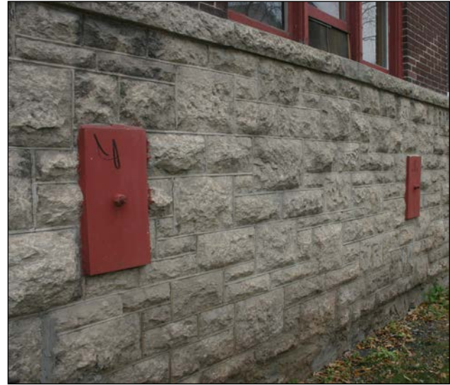
Left: Front (north) façade entrance detail; Right: Metal structural supports, 2009
