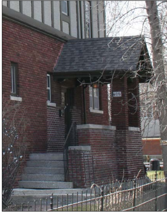
Side entrance detail, 2009
