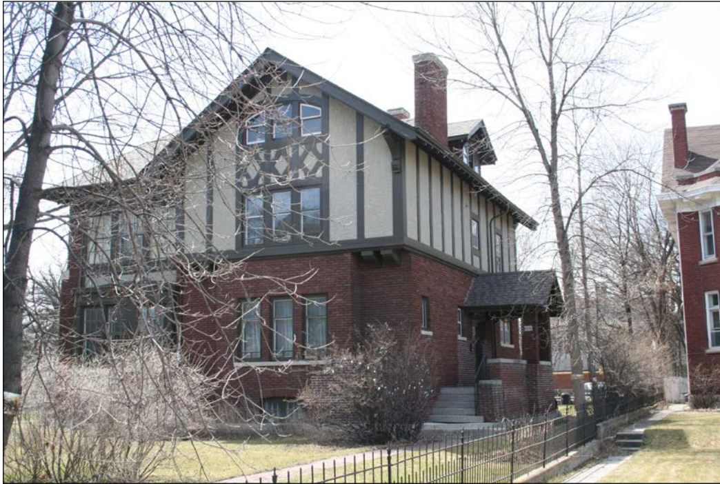
Front (east) and north façades, 2009
