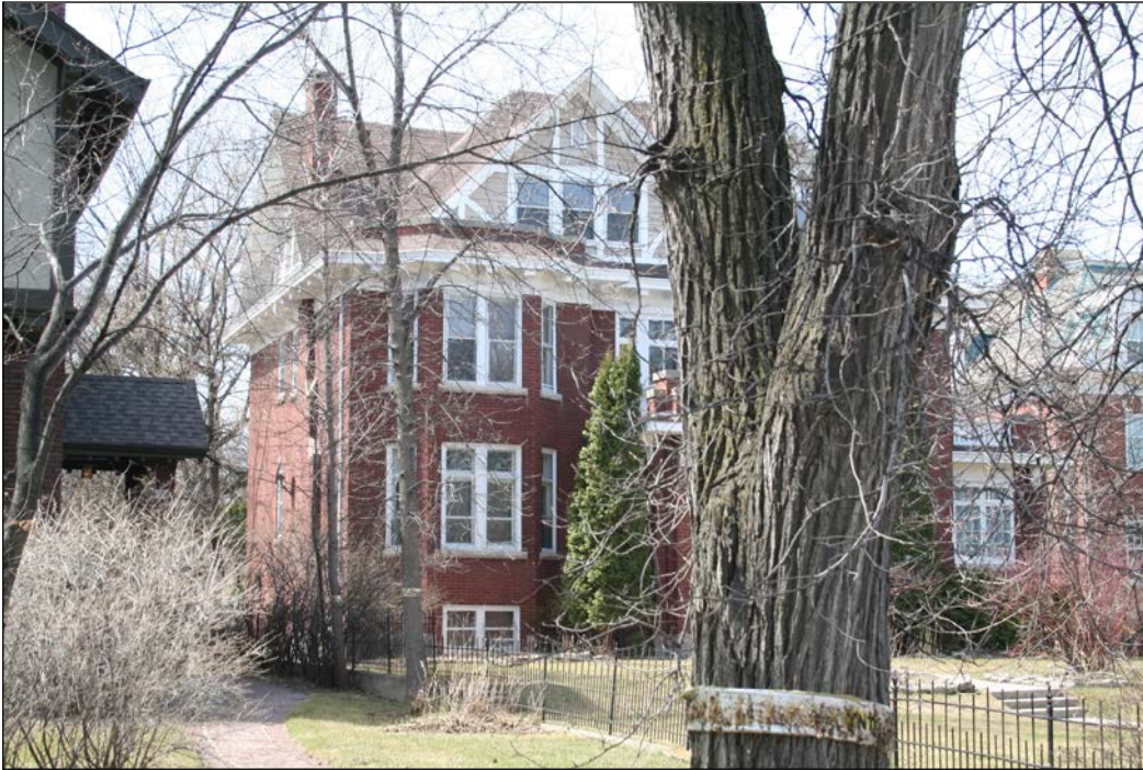
Front (east) and south façades, 2009
