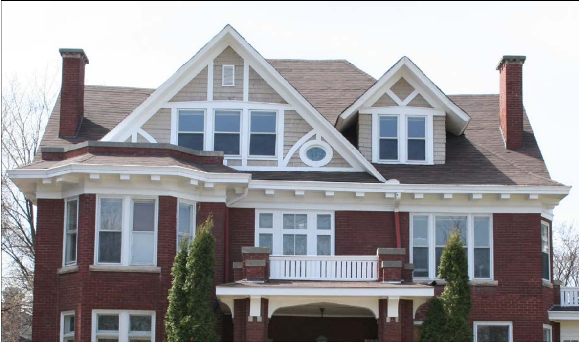
Front (east) façade roof detail, 2009
