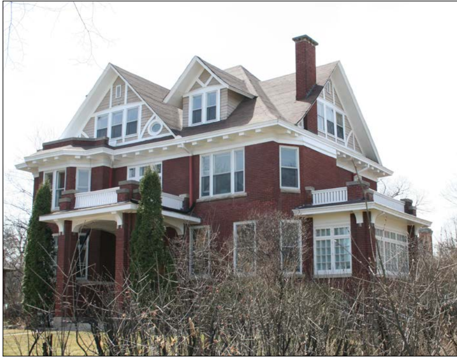
Front (east) and north façades, 2009
