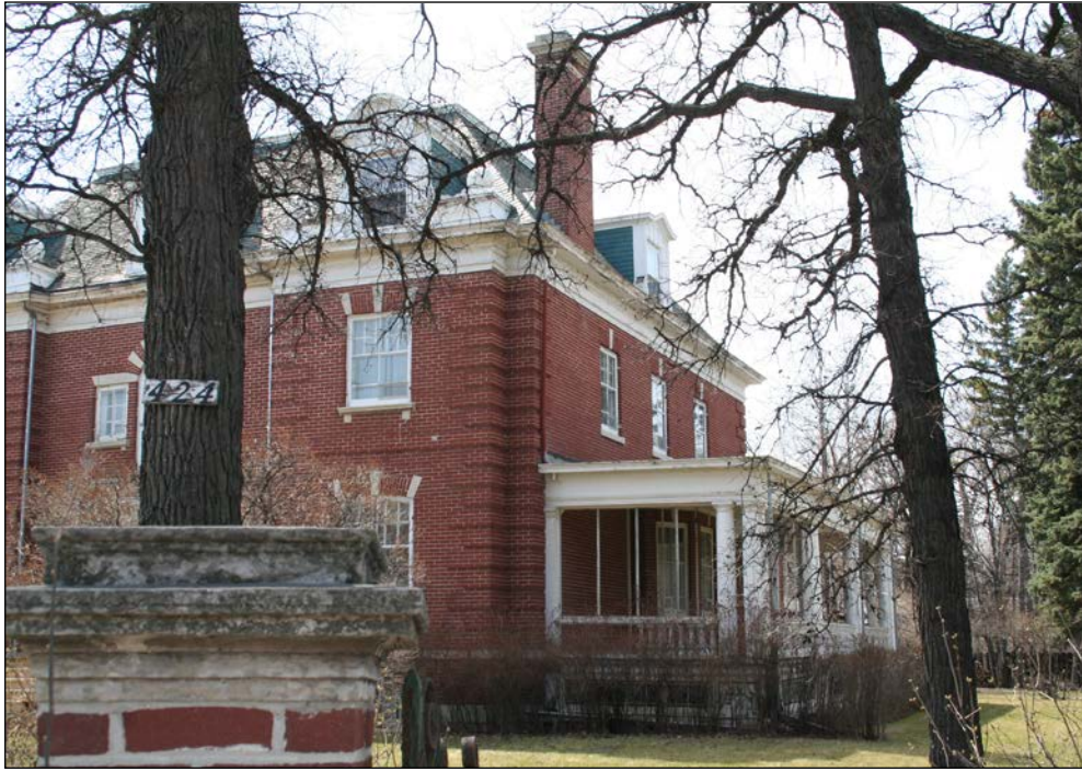
Front (east) and north façades, 2009
