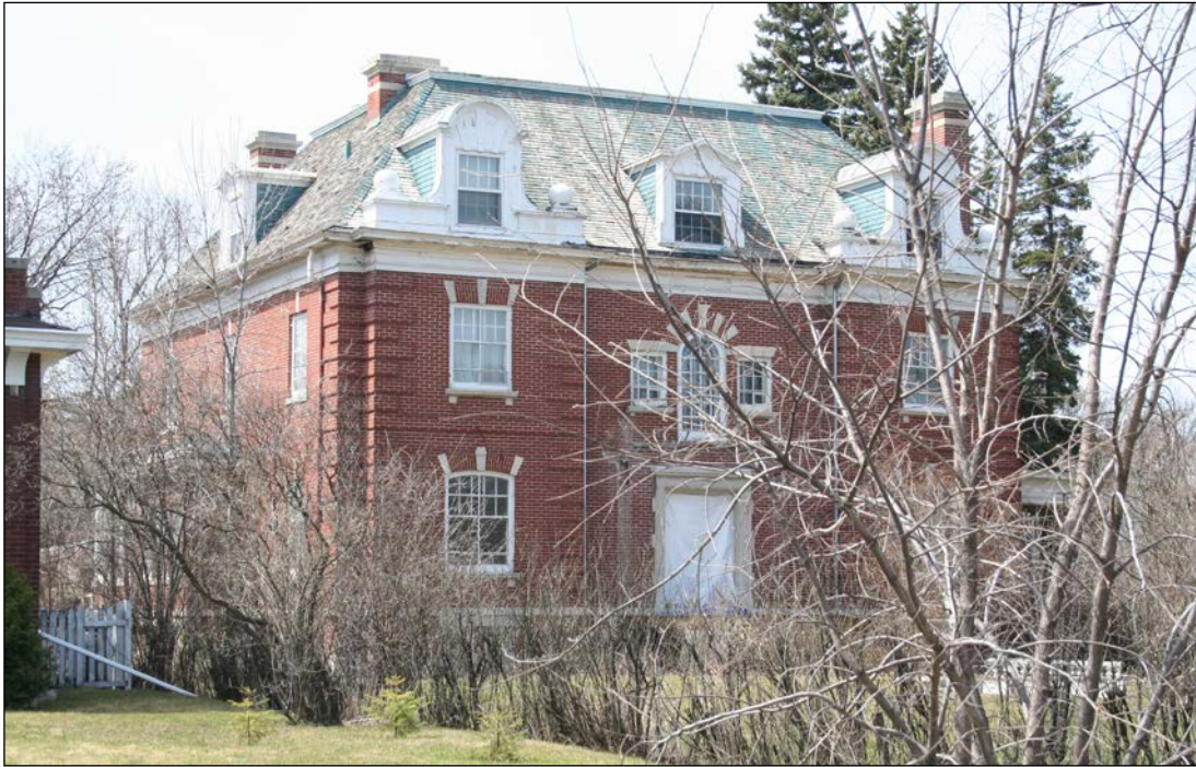
Front (east) and south façades, 2009
