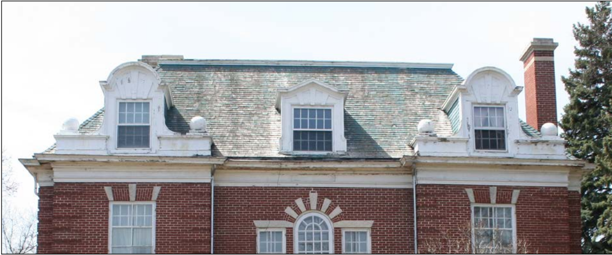
Front (east) façade detail, 2009
