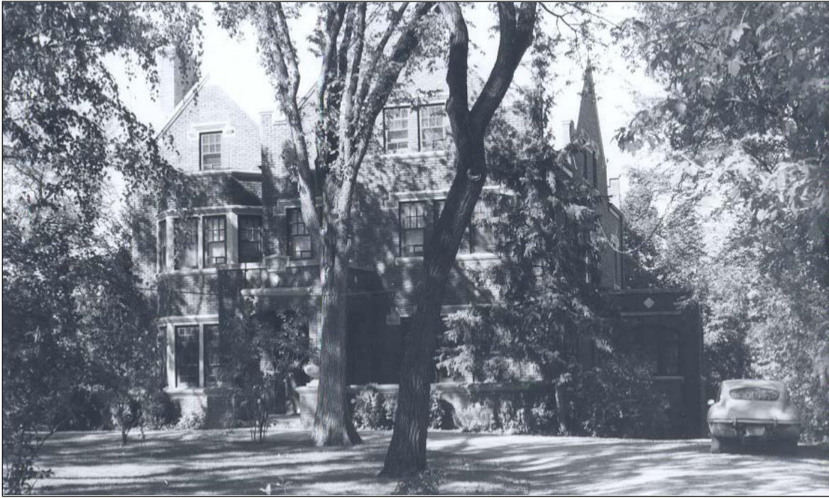
Front (south) façade, 1978
