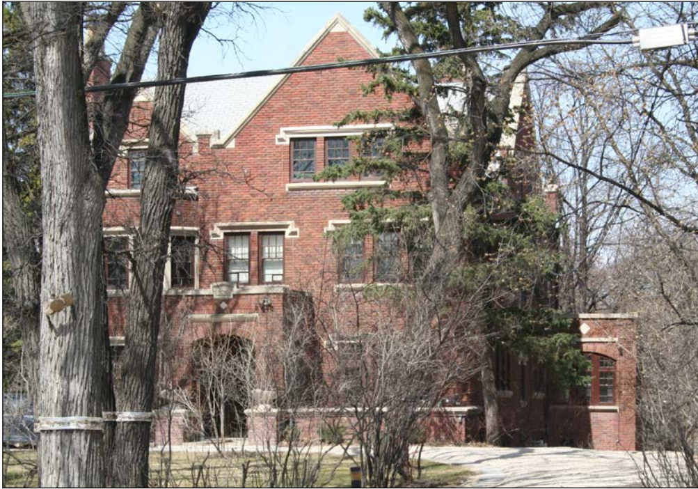
Front (south) and east façades, 2009
