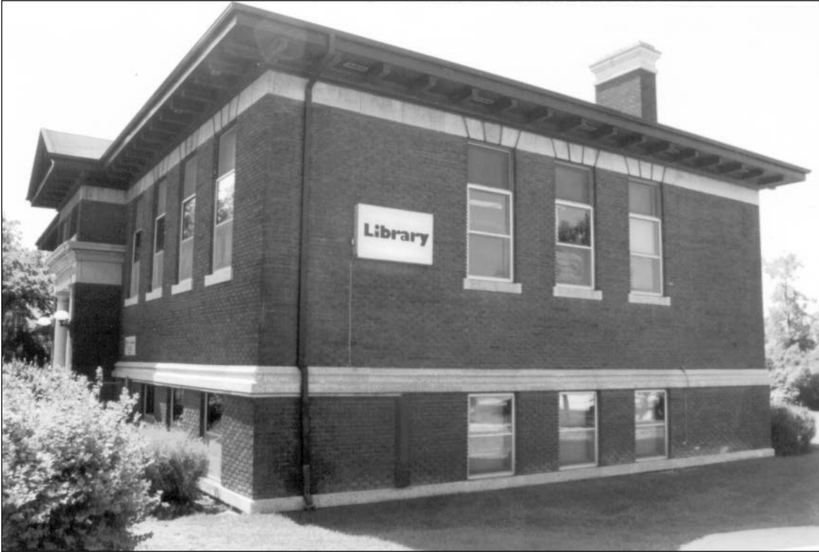
Plate 7 – Cornish Library, 20 West Gate, north façade. (M. Peterson, 1992.)
