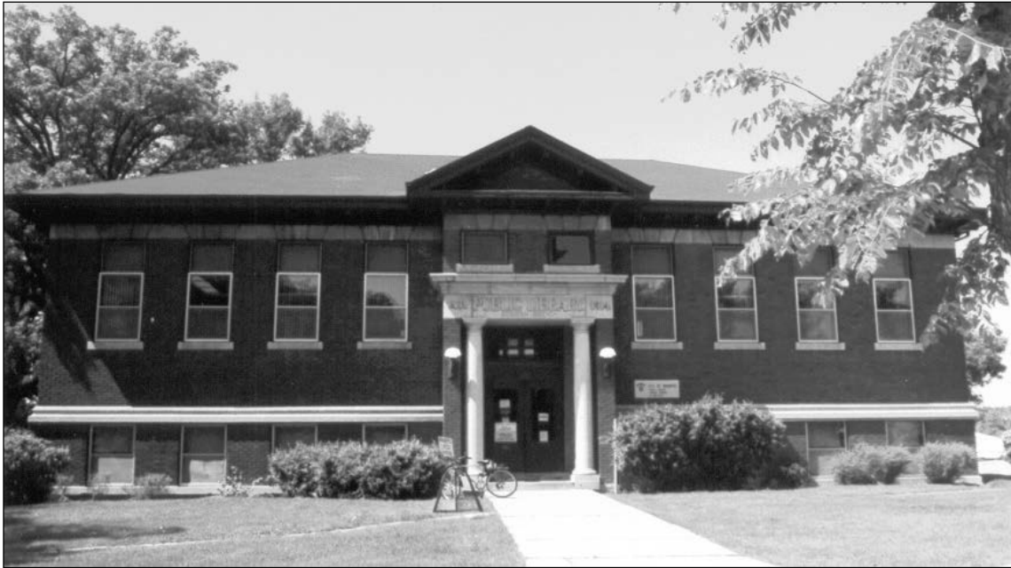
Plate 5 – Cornish Library, 20 West Gate; built 1914-15, architect S.F. Peters, National Construction Company, contractors; front or east façade. ( M. Peterson, 1992. )
