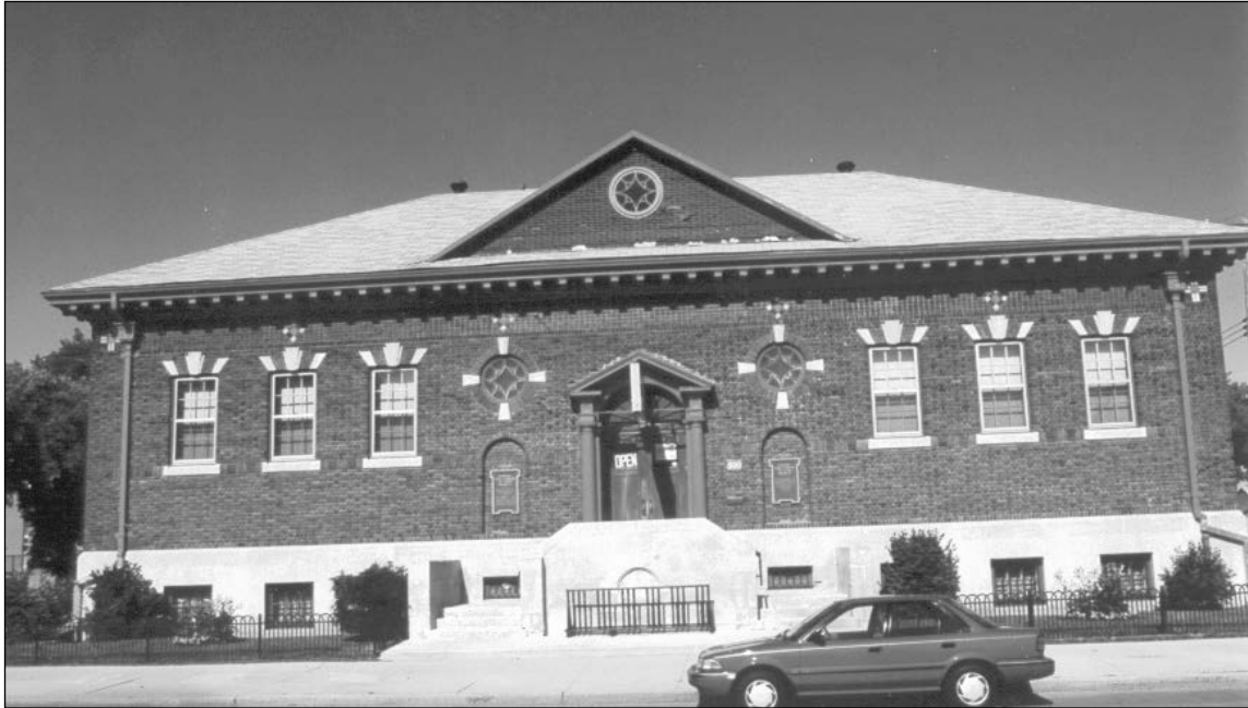
Plate 3 – St. John's Branch, 500 Salter Street; built 1914-15, architect J.N. Semmens, contractor Fraser and McDonald; front or east façade. (M. Peterson, 1992.)
