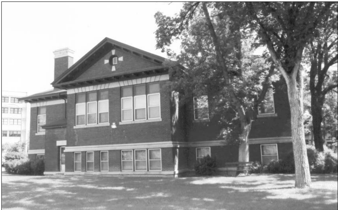
Plate 6 – Cornish Library, 20 West Gate, rear or west façade. ( M. Peterson, 1992. )
