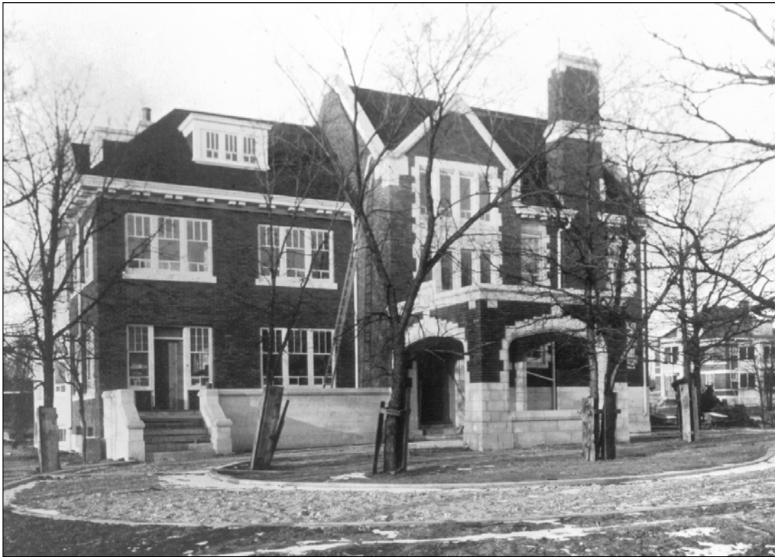
Plate 1 – R. Connor House, 54 West Gate during construction in 1914. This is the carriage entrance, now removed, on the east side. (Courtesy of the Provincial Archives of Manitoba.)
