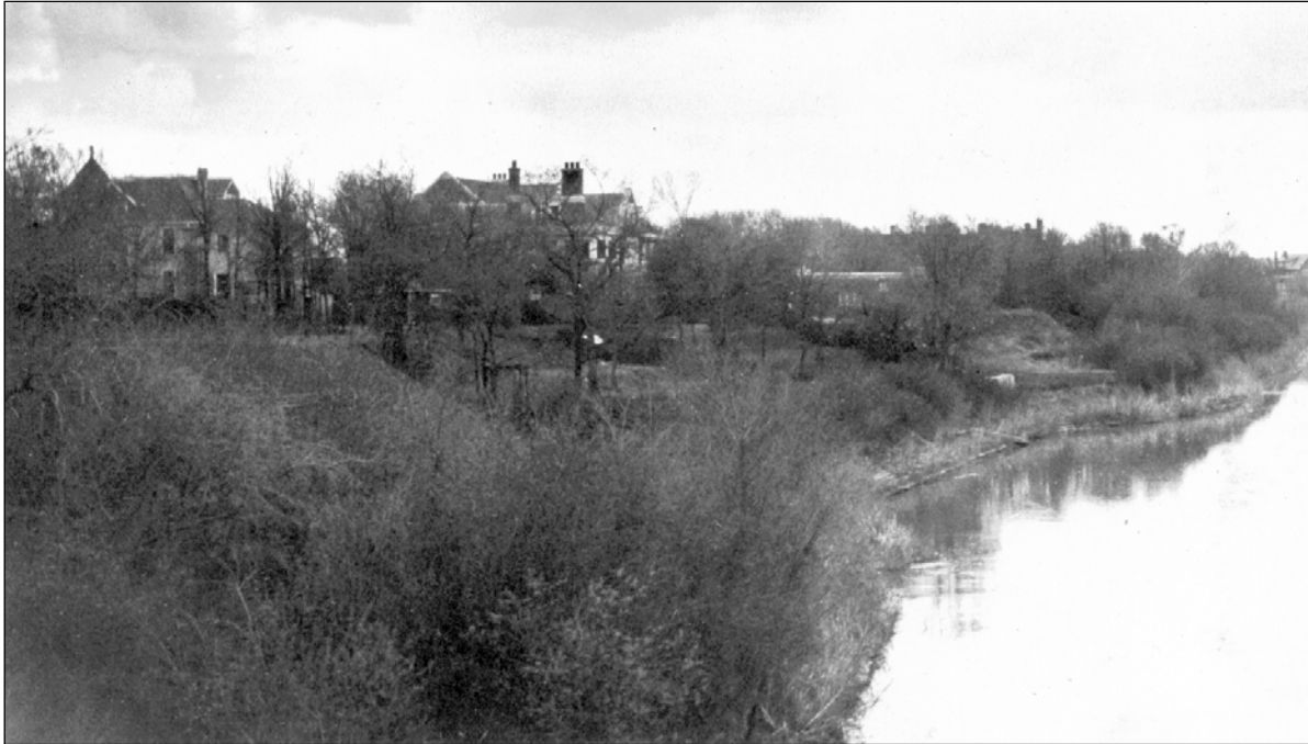
Plate 3 – 54 Westgate from where the Maryland Bridges now stand, ca.1915. (Courtesy of the Provincial Archives of Manitoba.)
