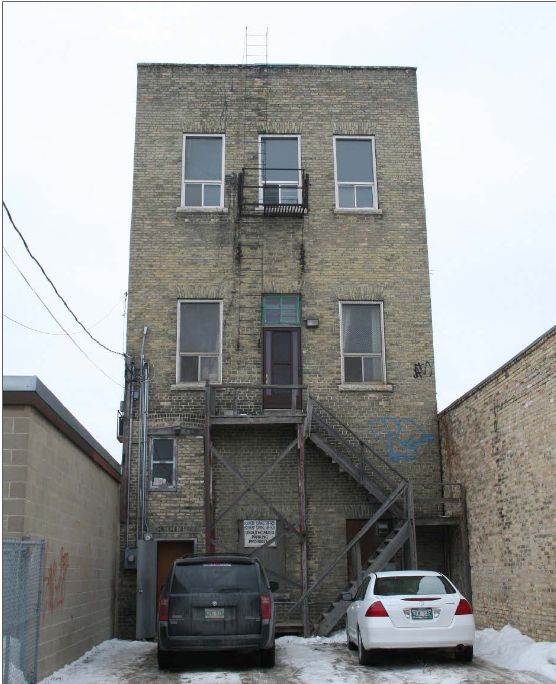
Plate 10 – Lauzon Block, 339 William Avenue, front (south) and east façades, 2014. ( M. Peterson, 2014. )
