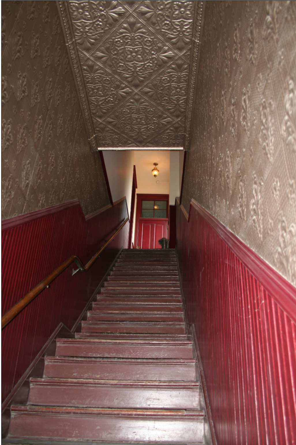
Plate 13 – Lauzon Block, 339 William Avenue, east side stairs to upper floors, 2015. ( M. Peterson, 2015. )
