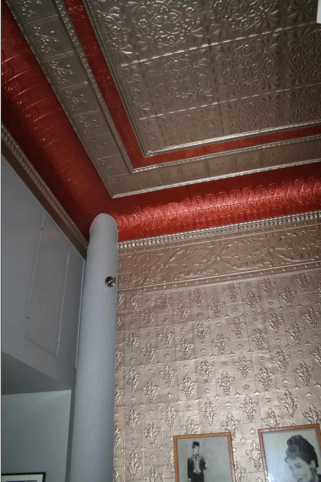
Plate 12 – Lauzon Block, 339 William Avenue, ground floor, refurbished ornamental tin, 2015. ( M. Peterson, 2015. )
