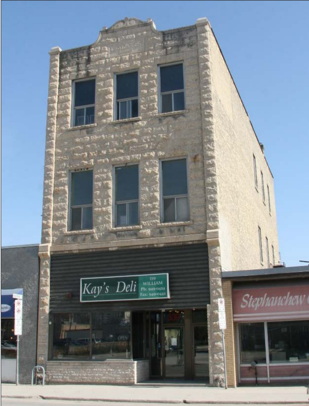
Plate 9 – Lauzon Block, 339 William Avenue, front (south) and east façades, 2015. ( M. Peterson, 2015. )
