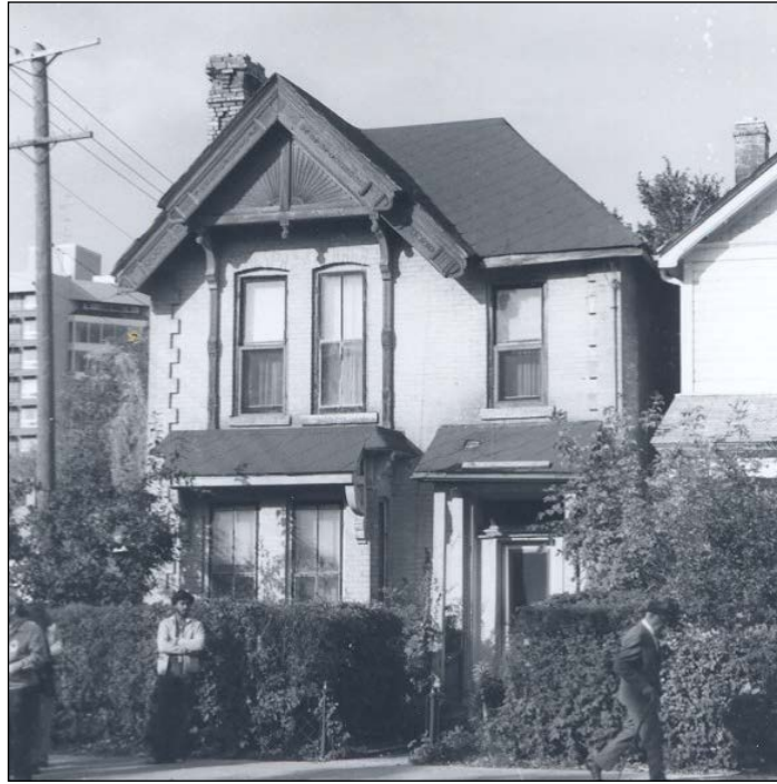
Front (south) façade, 1978
