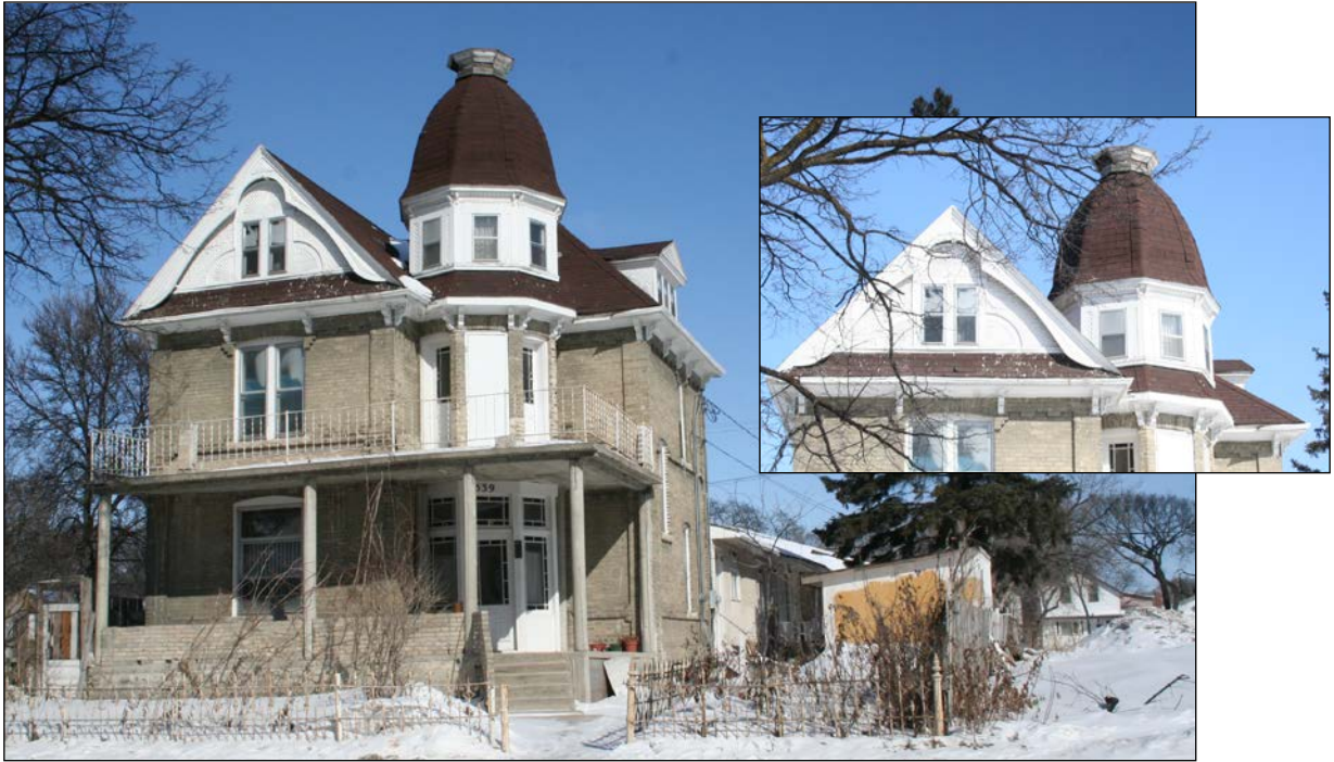
Front (south) and east façades and roof detail (inset), 2009
