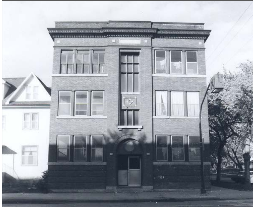
Front (south) façade, 1978
