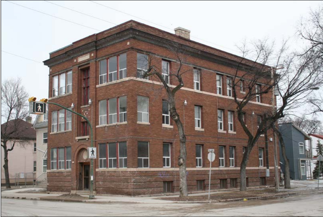
Front (south) and east façades, 2009
