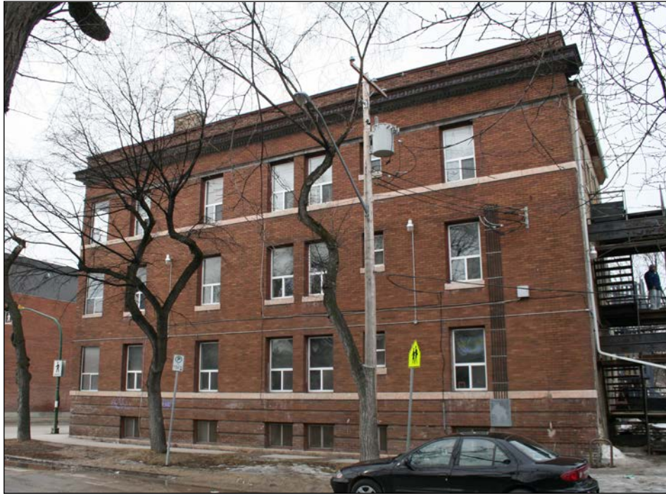
Rear (north) and east façades, 2009
