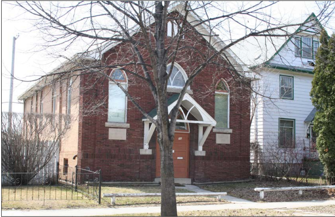
Front (north) and east façades, 2009
