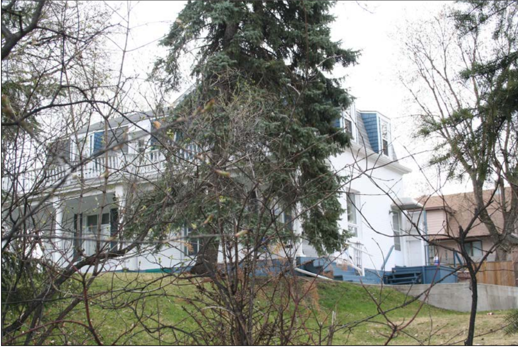
West and south façades, 2009
