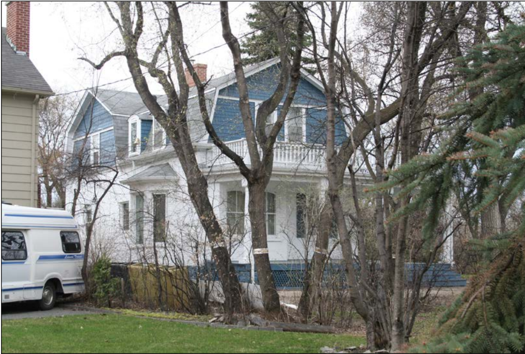
East and north façades, 2009
