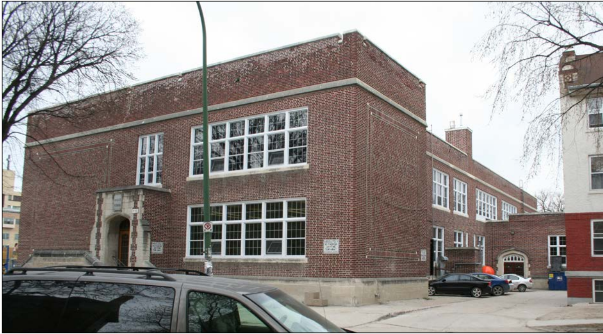
North and west façades, 2009
