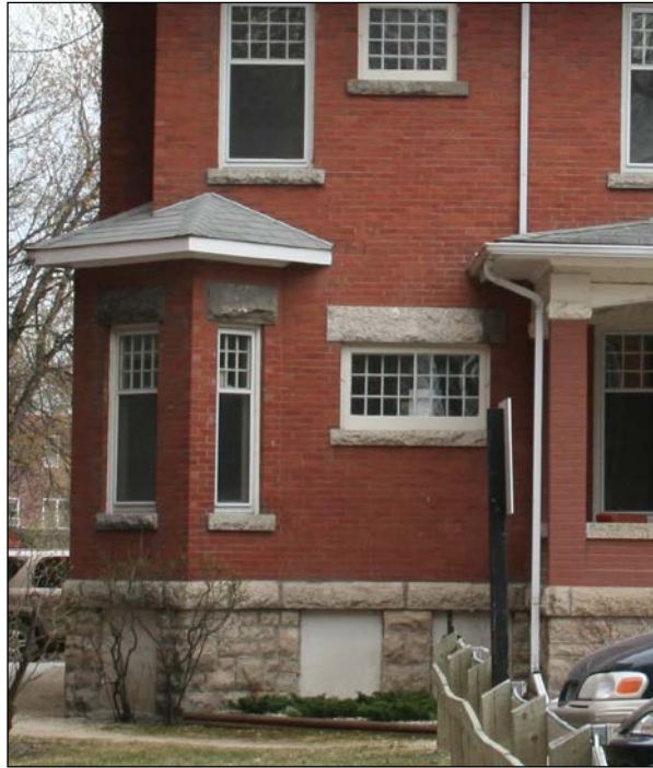
Northeast corner detail, 2009
