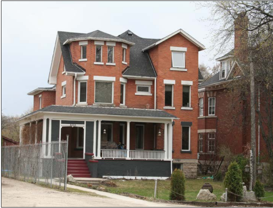
Front (north) and east façades, 2009
