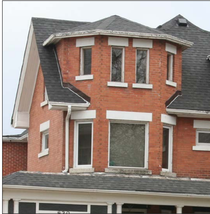
Northeast corner detail, 2009
