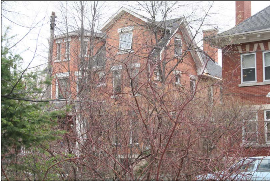
Front (north) and west façades, 2009
