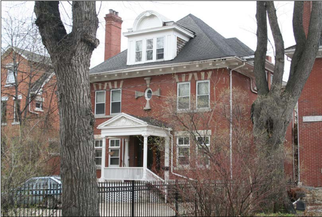
Front (north) and west façades, 2009
