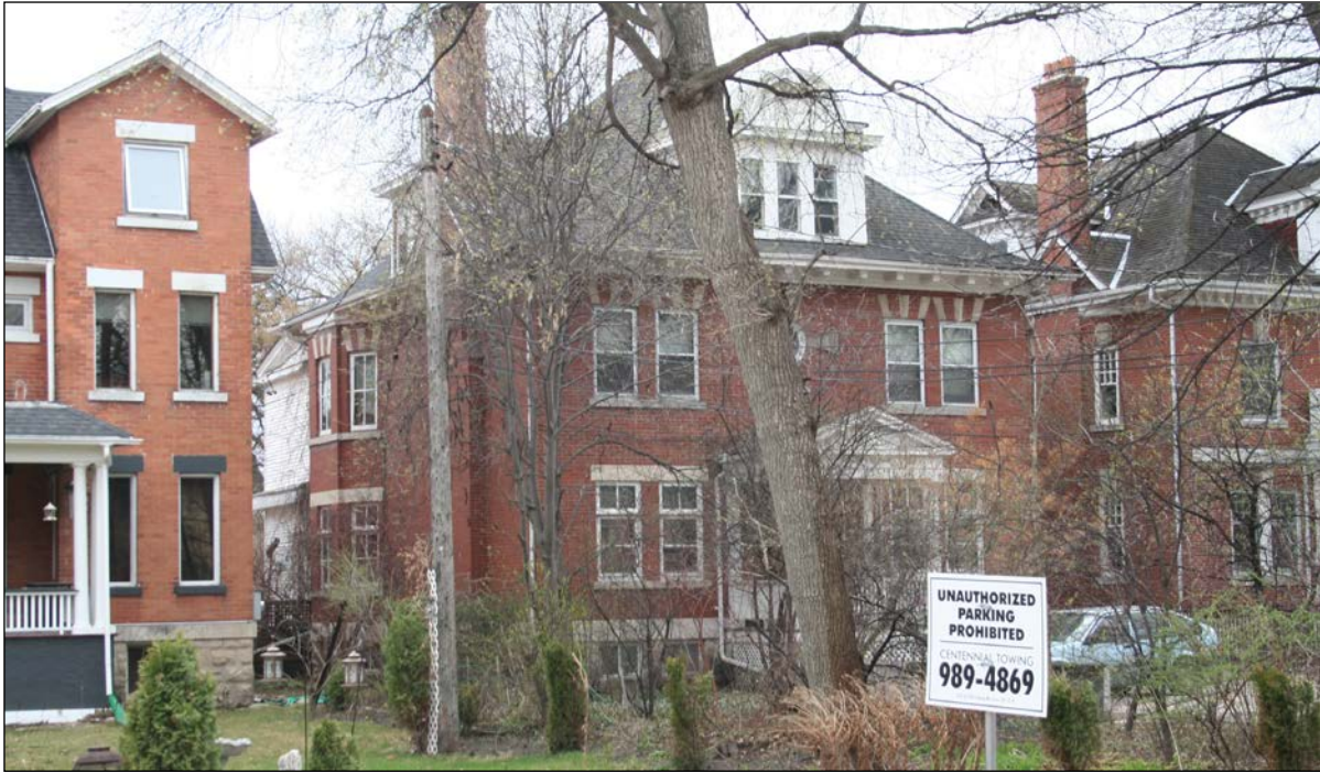
Front (north) and east façades, 2009
