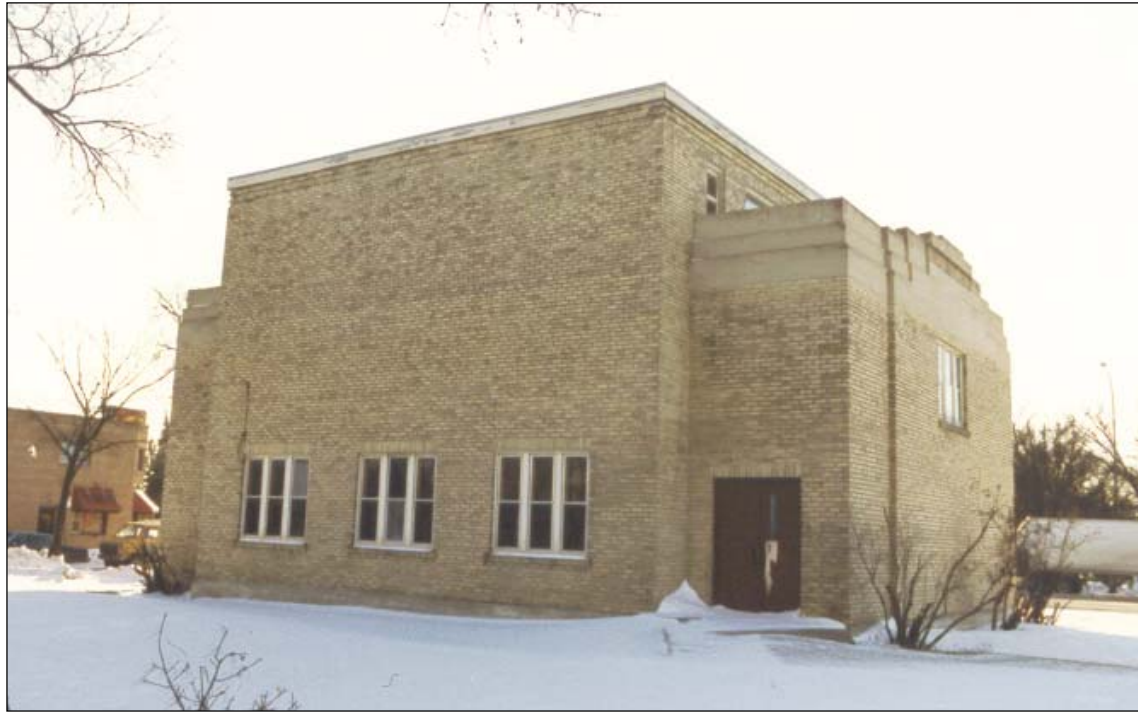
Plate 4 – Rear (west) and north façades, no date. (M. Peterson.)
