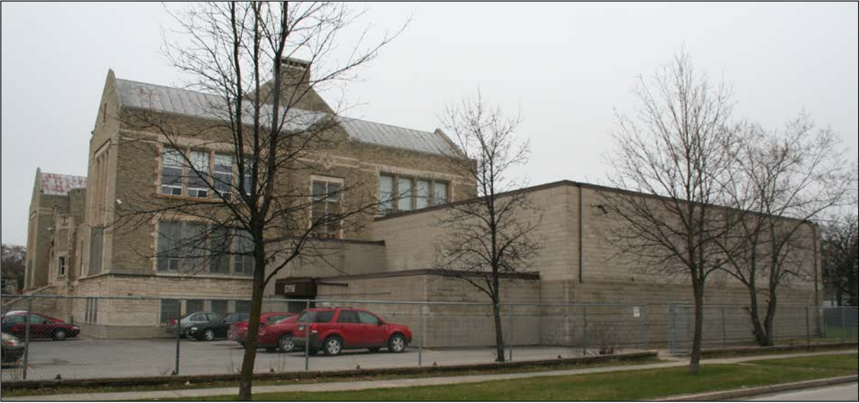
Front (east) and north façades, 2009
