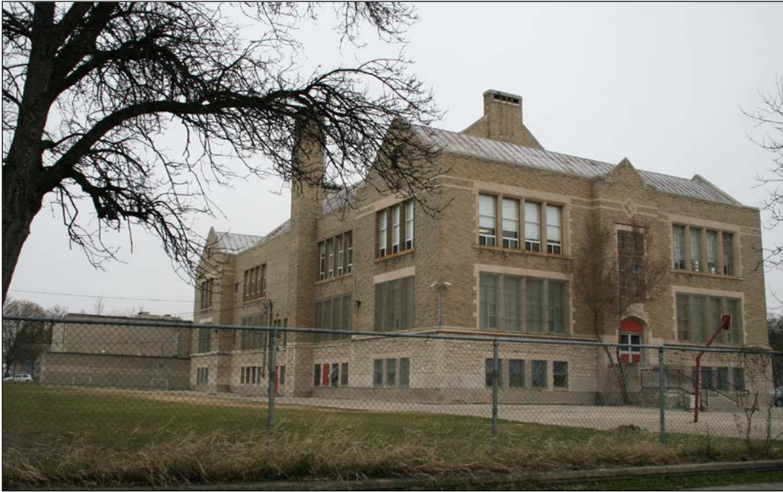
Rear (west) and south façades, 2009
